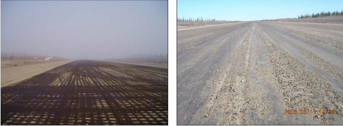
Figure 10. Example of non-uniform application and the result after 1 year (photo courtesy of ADOT&PF)
