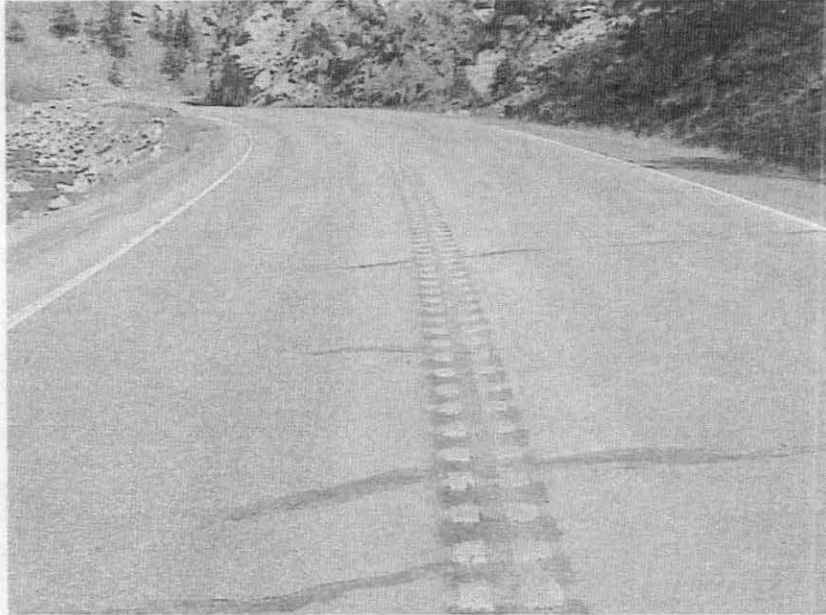
Figure 1. State Highway 119 in Boulder Canyon winds through Forest Service land.
