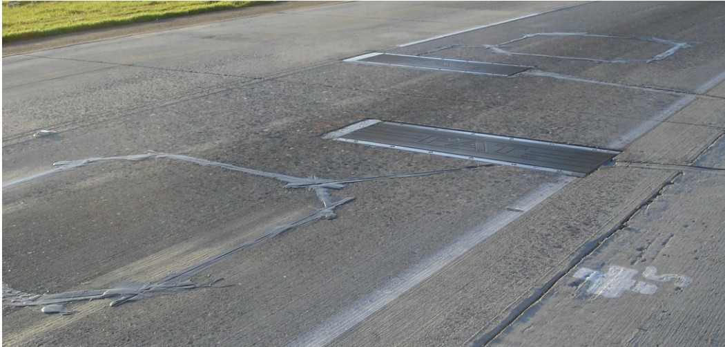
Figure 3. Photo. Staggered bending plate installation and inductive loops. (33)
