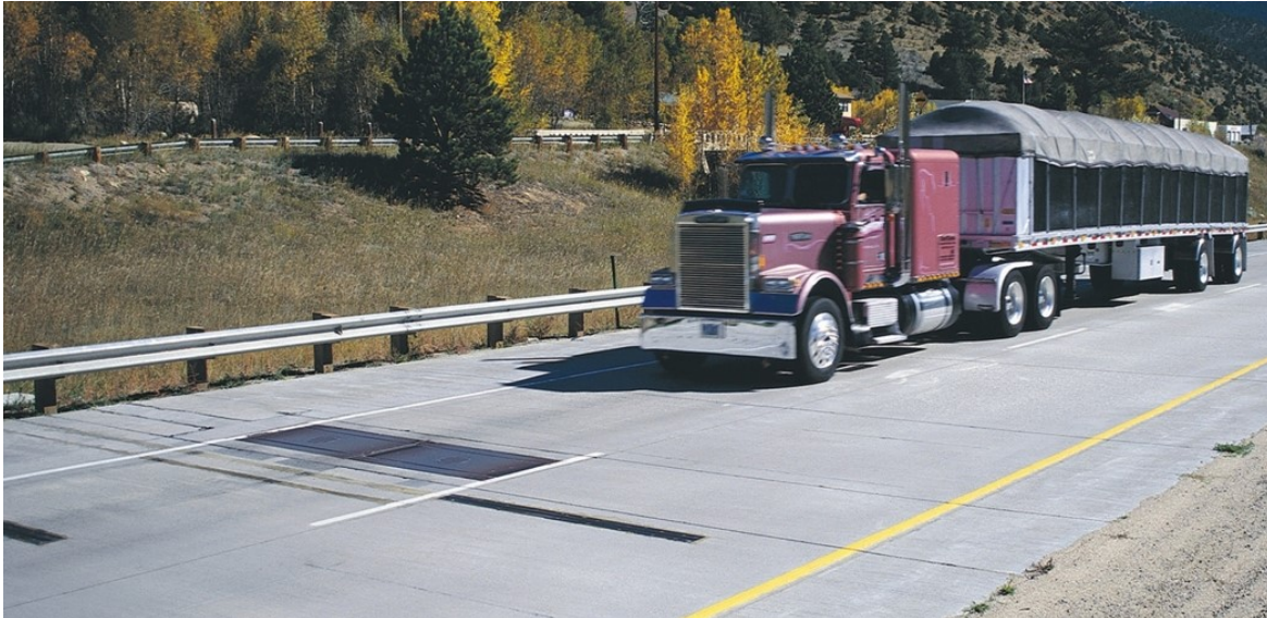
Figure 4. Photo. Inline configuration of load cell-based weight sensors. (33)
