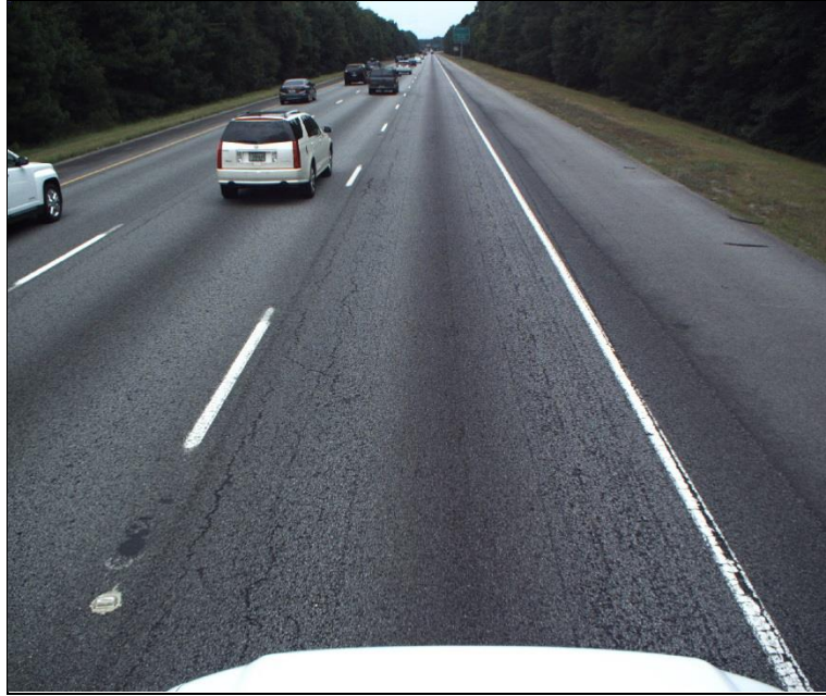
Figure 3.5 Photo taken on I-95 Northbound MP 13-14 Chatham County in 2014
