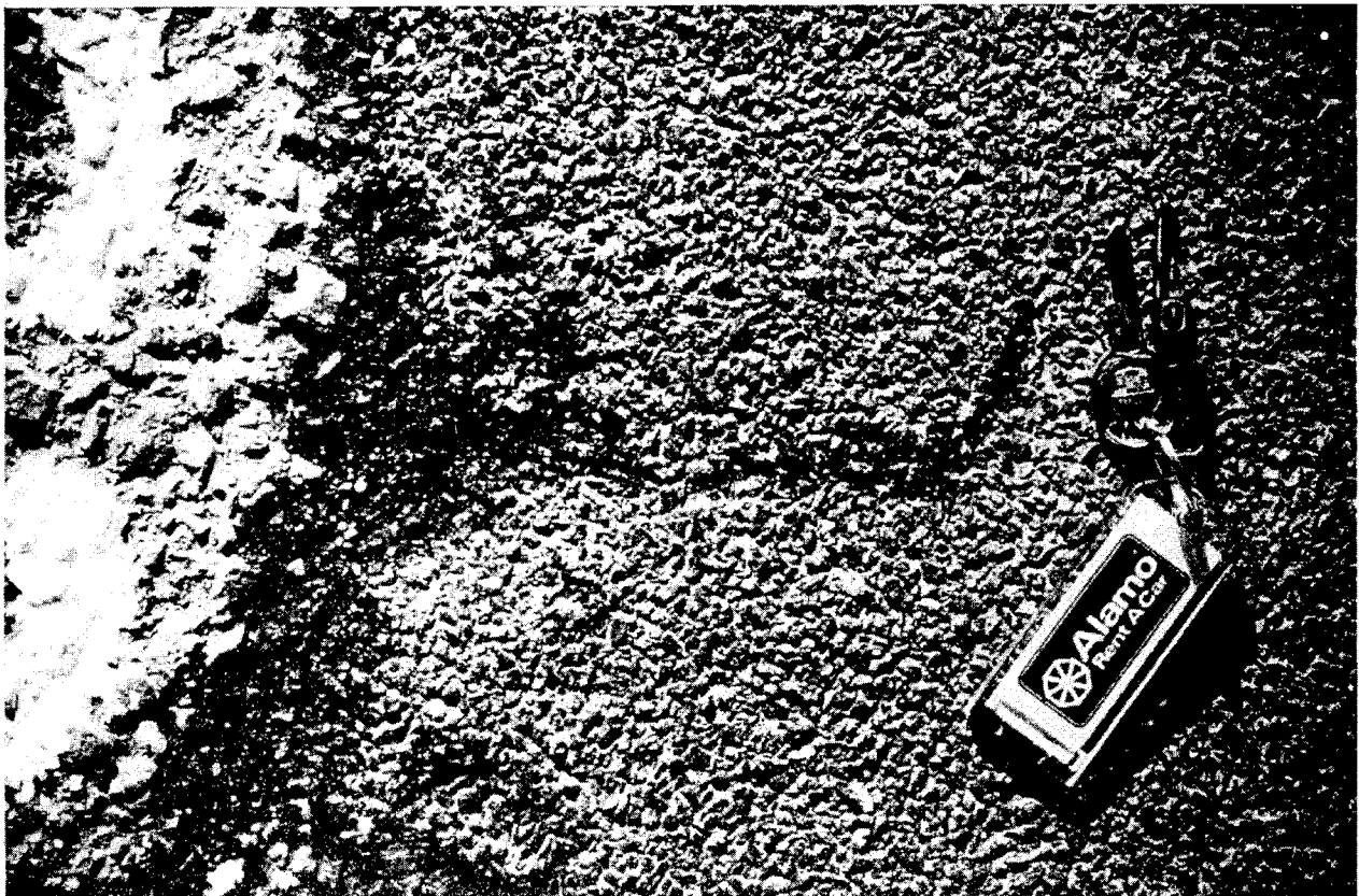
Figure 32. Example of cracking distress.
