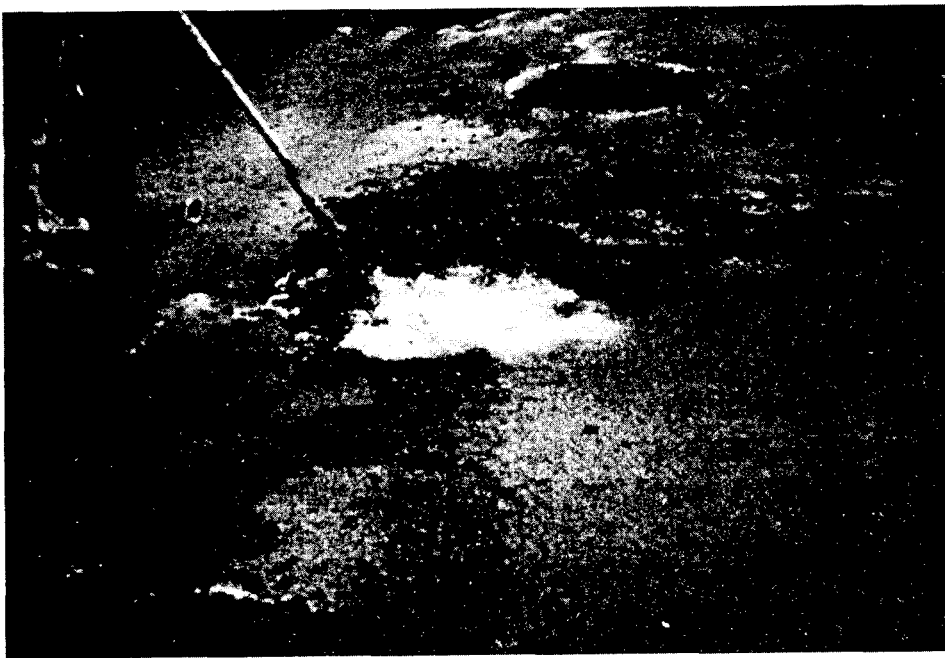
Figure 17. Heating cold mix with propane torch.
