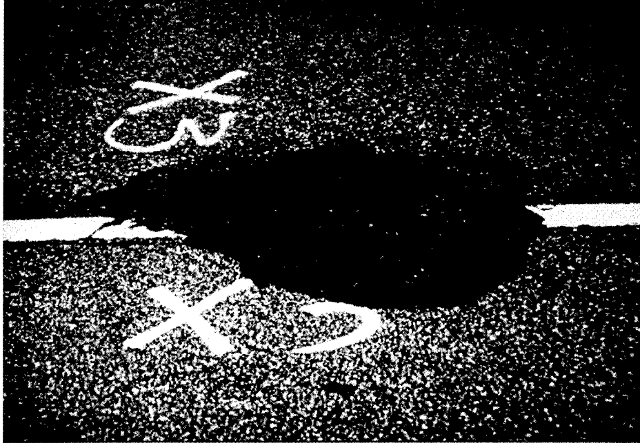
Figure 31. Example of shoving distress.
