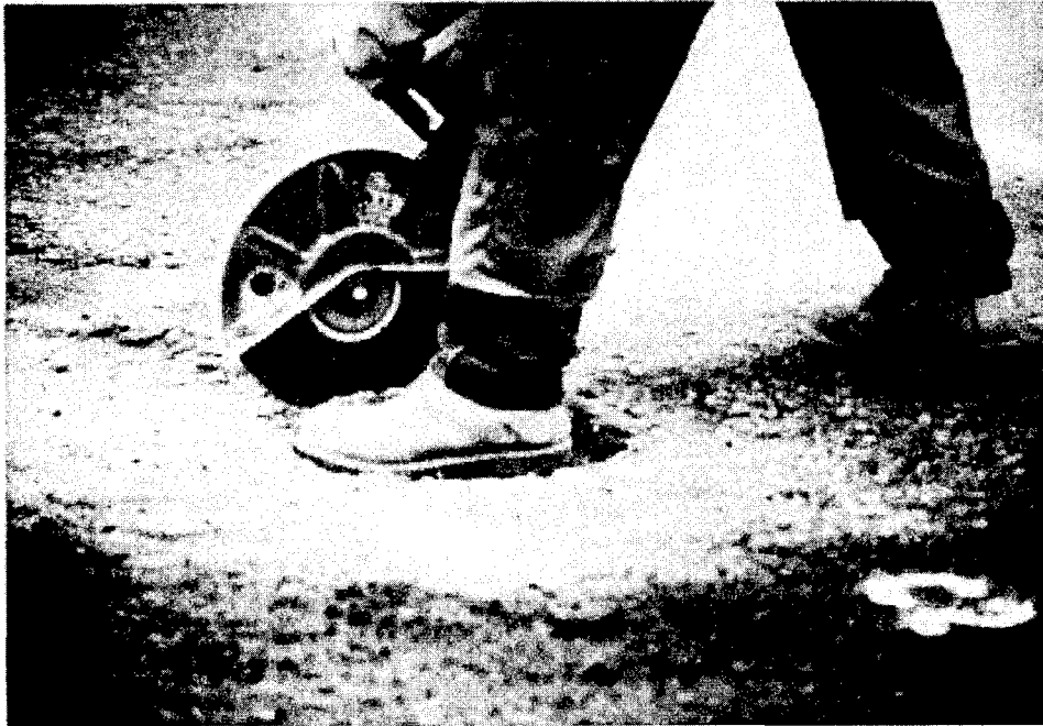
Figure 15. Straightening sides using pavement saw.
