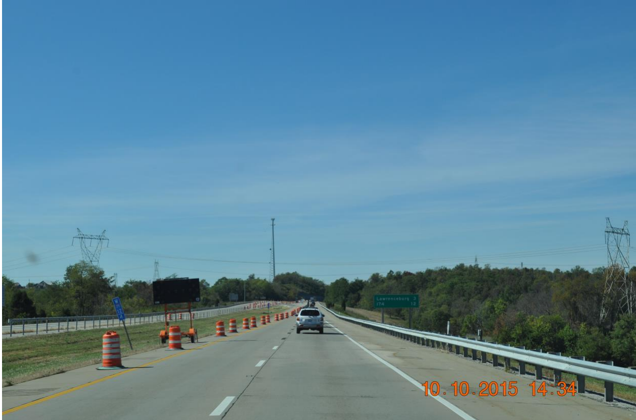
Figure 4 I-275 case study, merging point. Message board flashes arrow during peak traffic hours.
