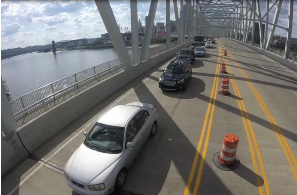
Figure 12 Snapshot from video of zipper merge in action on Taylor Southgate Bridge
