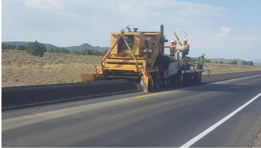
Figure 28. CIR construction on the Fernley CIR project.
