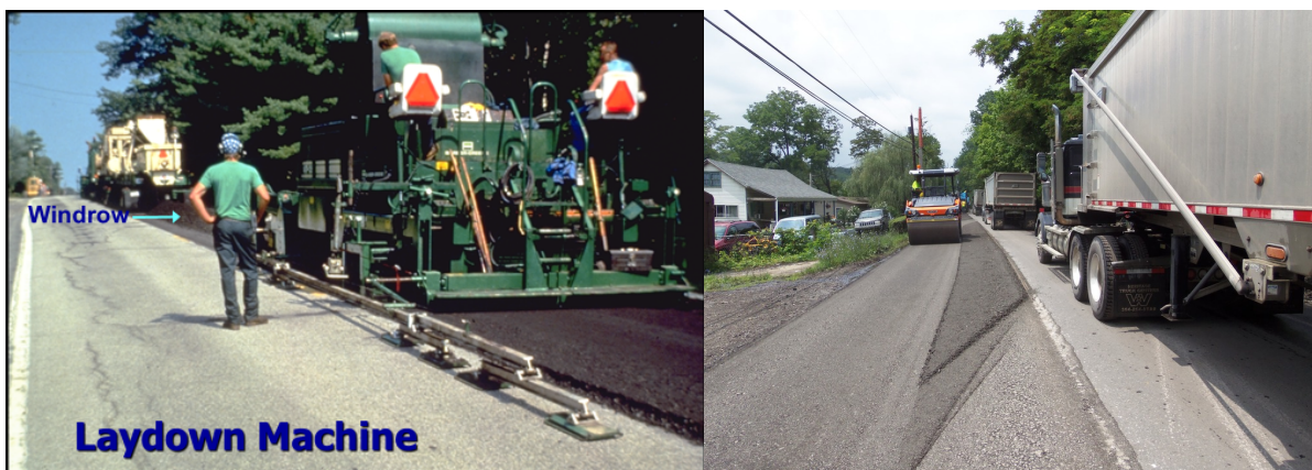
Figure 2. The CIR mix is picked up by the paver and roller compacted.
