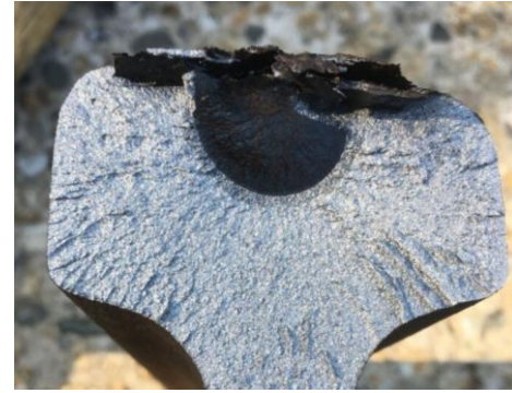
Figure 9: Transverse Defect and Potential Electrode Pitting in Rail Head
