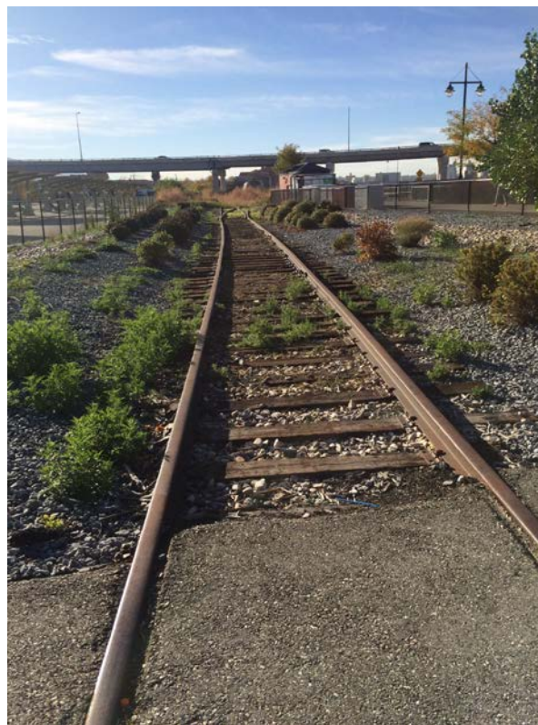
Figure 5.1 FrontRunner corridor under highway infrastructure
