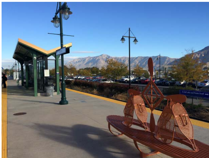
Figure 1.4 Park-and-ride facility next to a FrontRunner station
