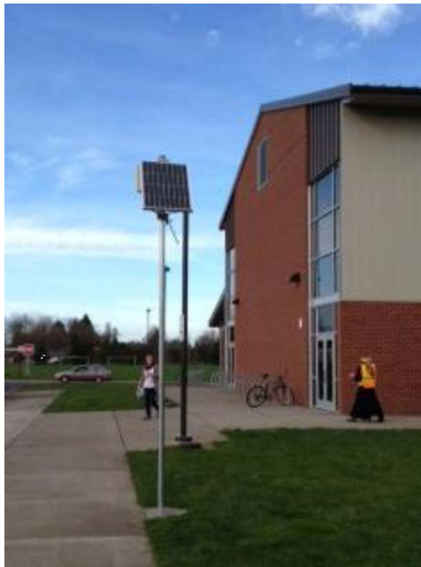
Figure 4.2: A Boltage Device Installed at One of the Experimental Schools
