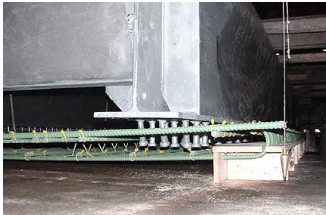
Figure 9: Prefabricated Bridge Units cast Upside-Down (Fort Miller Company 2016)
