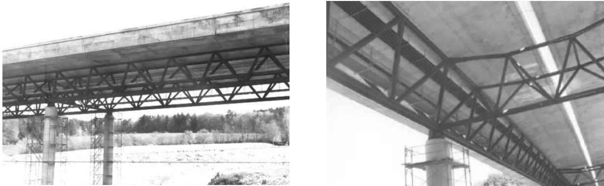
Figure 14: Lully Viaduct Space Truss ((Dauner et al. 1998))
