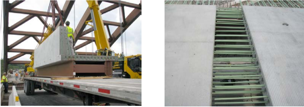
Figure 10: I-87 Prefabricated Bridge Unit Installation, I-87 Bridge Reconstruction (Fort Miller Company 2016)
