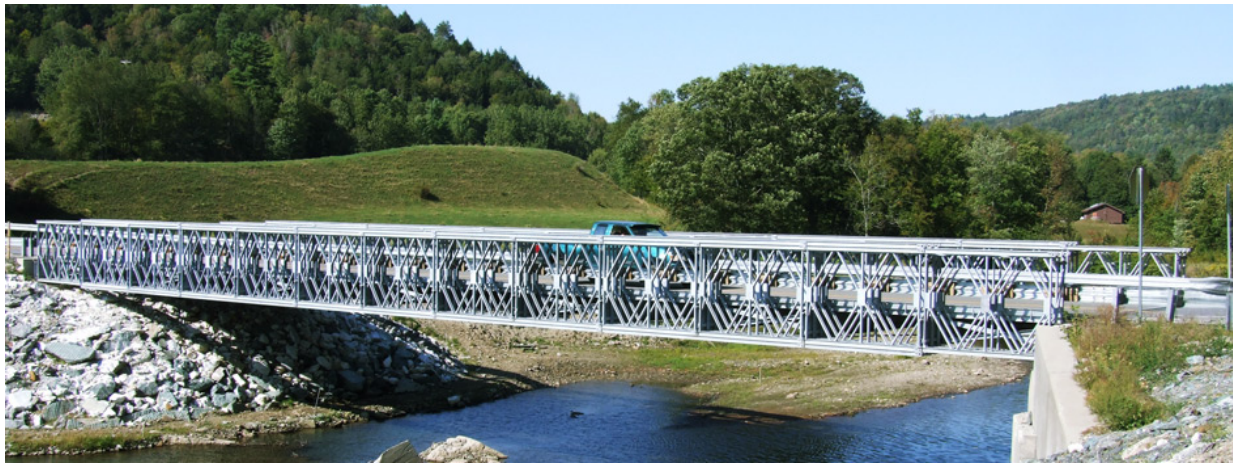
Figure 5: Acrow Bridge assembled using Several Layers of Panels to Achieve the Span (Acrow Corporation of America 2015)
