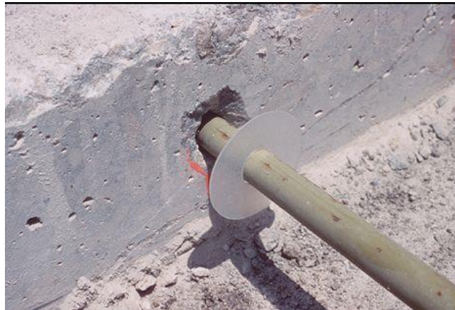
Figure 22. Grout retaining disk. (Photo Courtesy of Mark B. Snyder)
