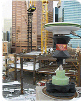
Photo courtesy of WSP Canada Inc GPS HPR receiver used in construction/surveying
