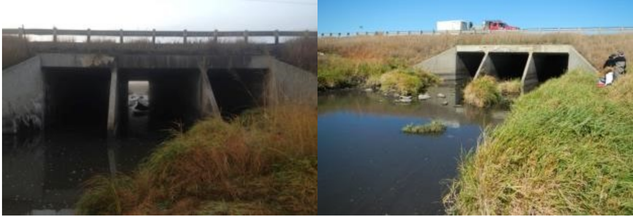
Figure 2.4 Upstream view of culvert 91077 on Elk Creek, Rock County, showing a portion of the small pool (left) and downstream view of culvert 91077, showing vegetated islands and rip-rapped area.
