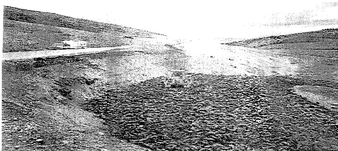
Figure 7. Lightweight tire fill under construction over the spring box culvert.
