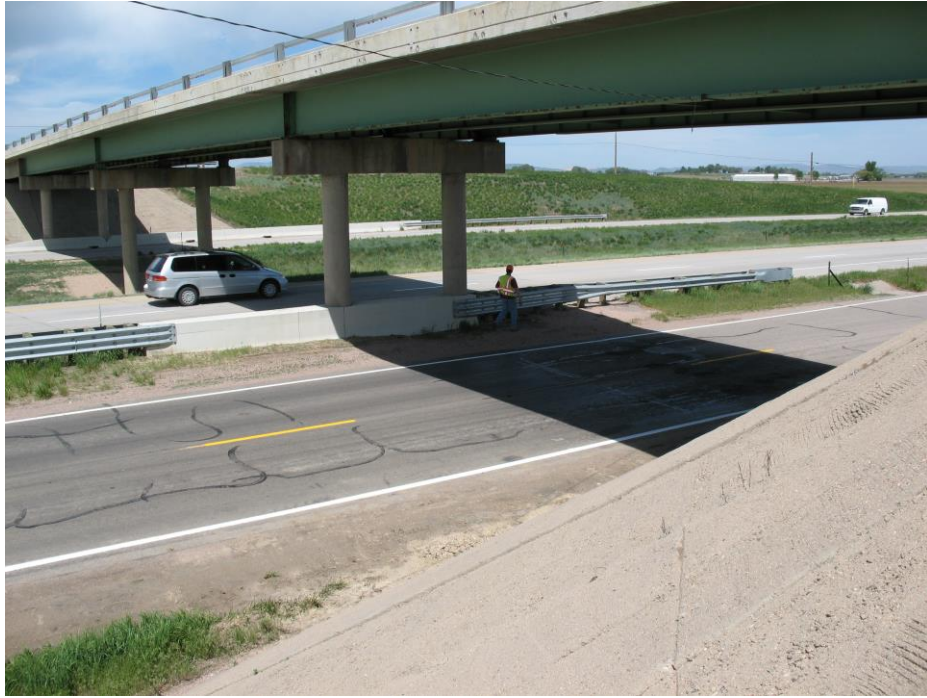
Figure 3-3. View of B-16-FM from East Abutment (Photo courtesy of CDOT)
