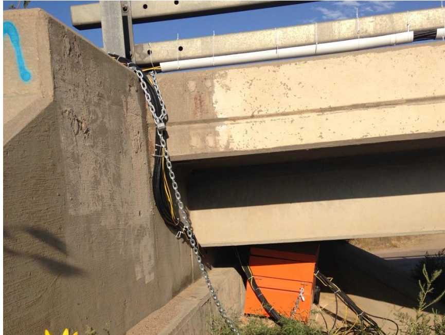
Figure 3-25 Job Box on North Abutment'
