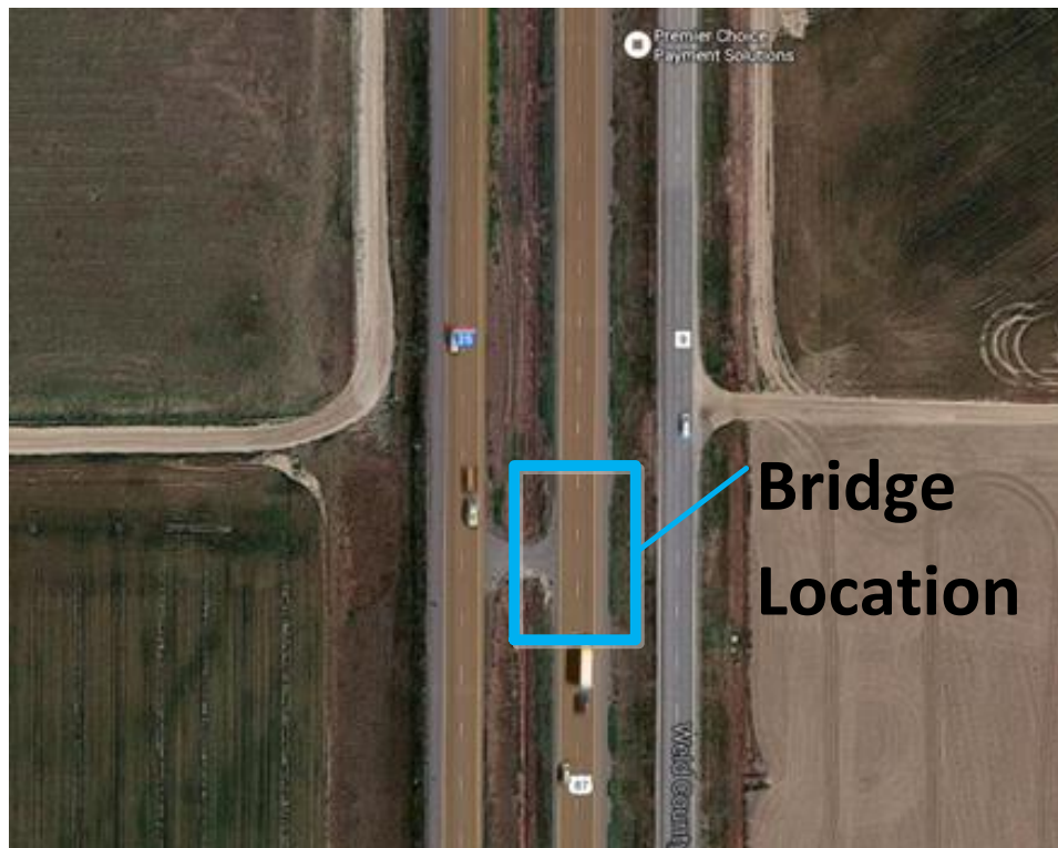
Figure 3-5. Aerial View of C-17-AT (Photo courtesy CDOT)
