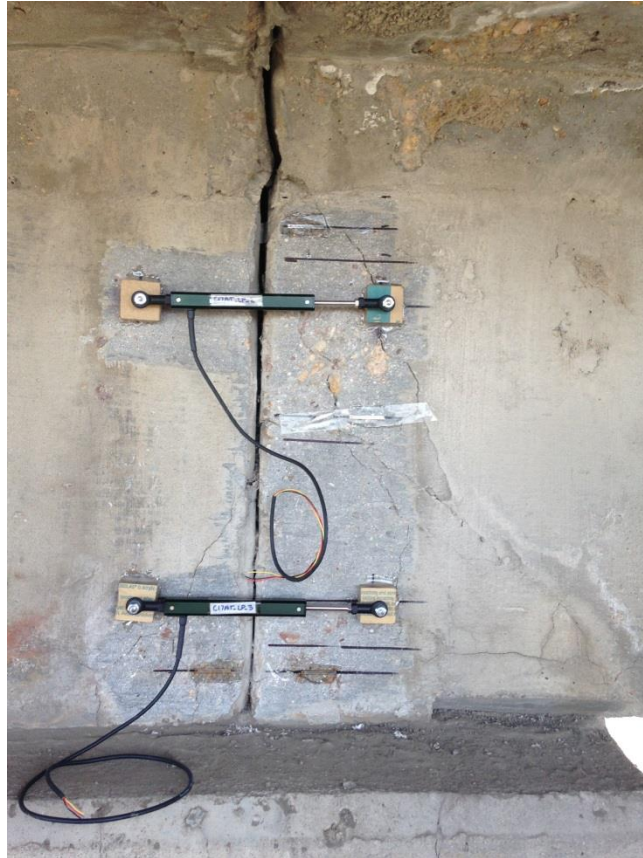
Figure 3-21 Linear Potentiometer in Place on Joint
