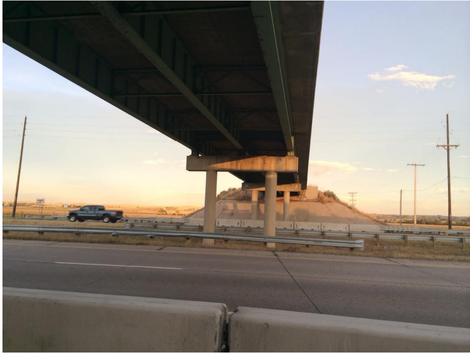
Figure 3-2. B-16-FM Superstructure from the West Abutment (photo by Authors)
