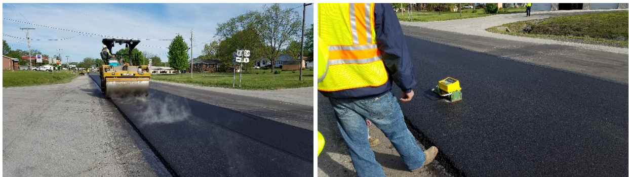
Figure 31: Trial Section Tests on 4/24/2017 (J1P3005 RT 24).
