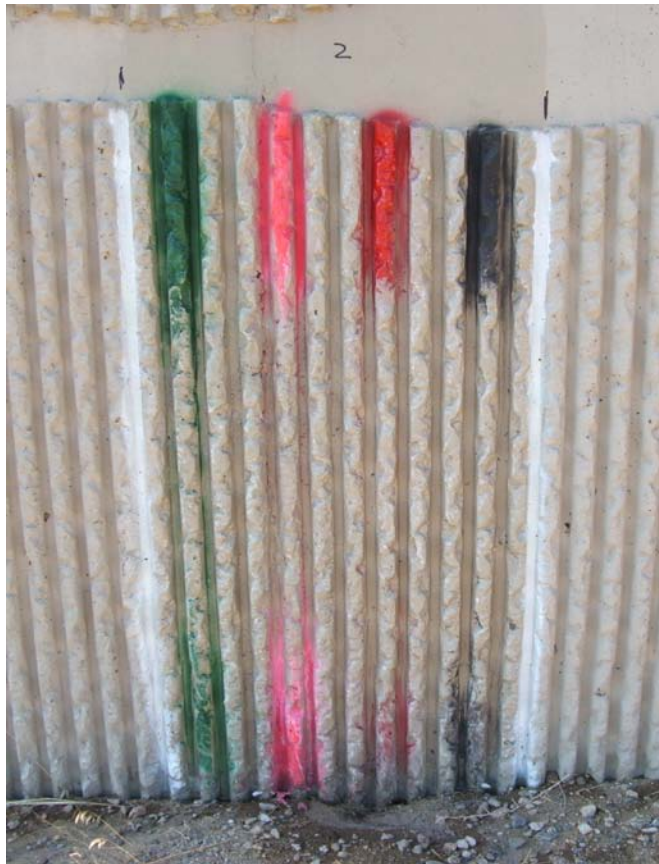
FIGURE 4.2C Removal - Fractured Fin Facing Panel 2
