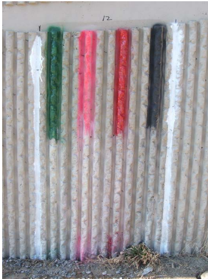
FIGURE 4.12C Removal - Fractured Fin Facing Panel 12
