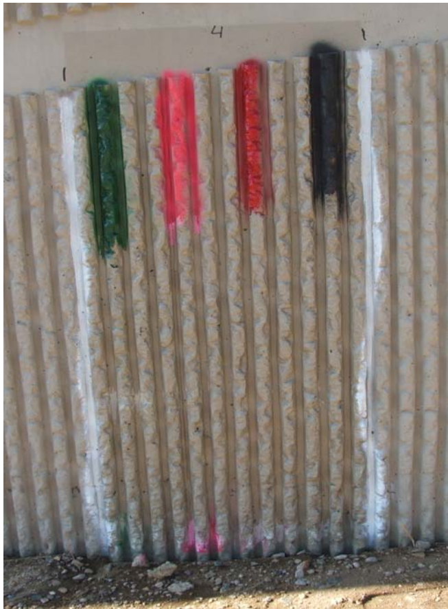
FIGURE 4.4C Removal - Fractured Fin Facing Panel 4
