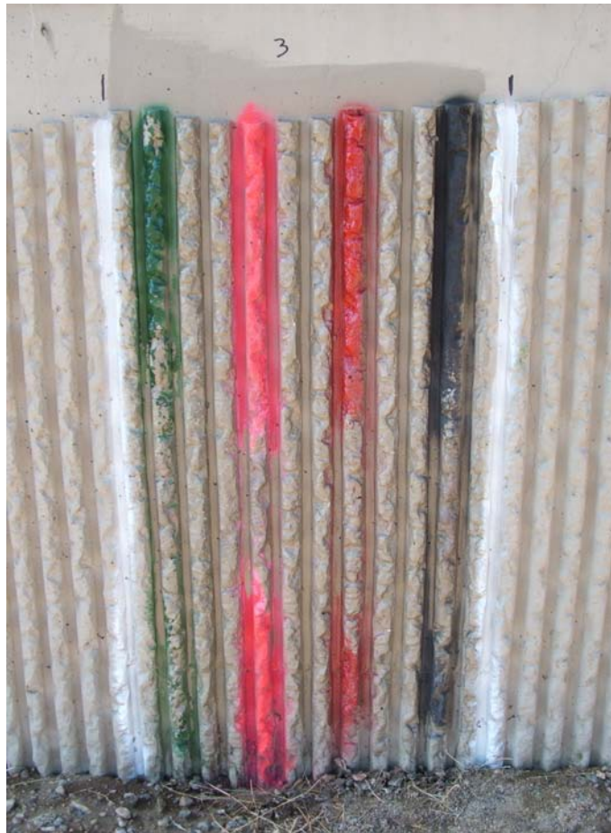
FIGURE 4.3C Removal - Fractured Fin Facing Panel 3
