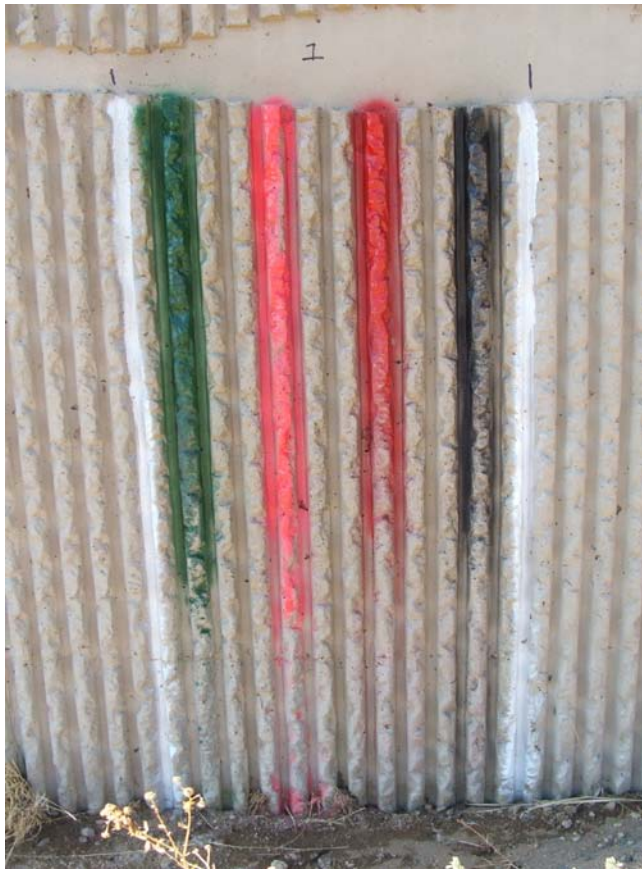
FIGURE 4.1C Removal - Fractured Fin Facing Panel 1
