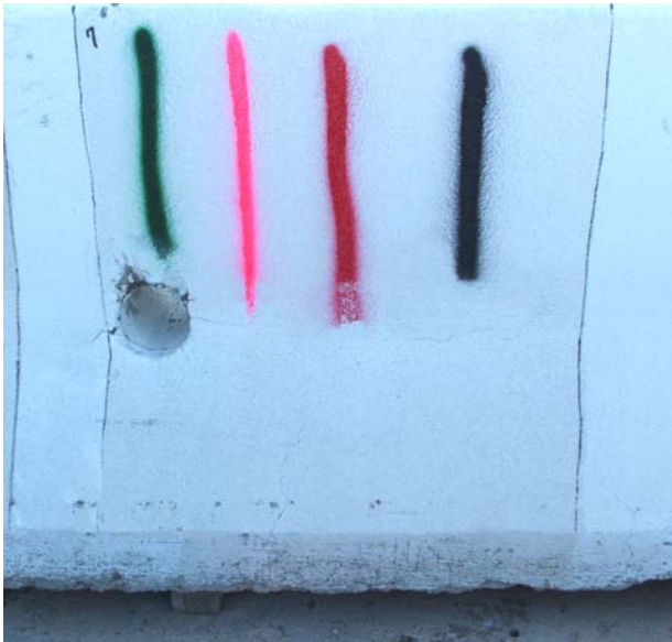
FIGURE 4.7A Removal - Painted Panel 7
