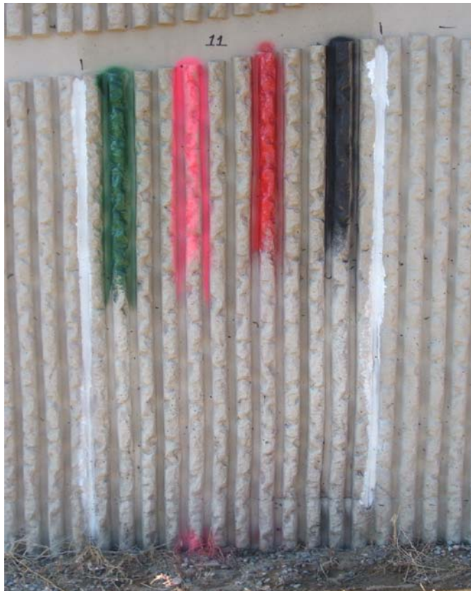
FIGURE 4.11C Removal - Fractured Fin Facing Panel 11
