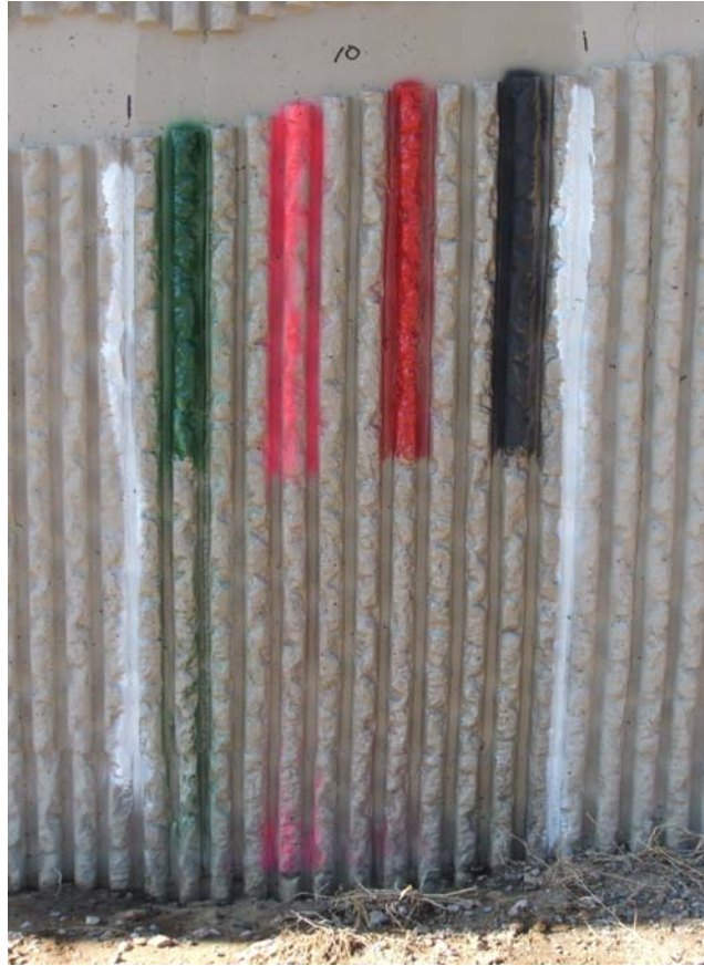
FIGURE 4.10C Removal - Fractured Fin Facing Panel 10
