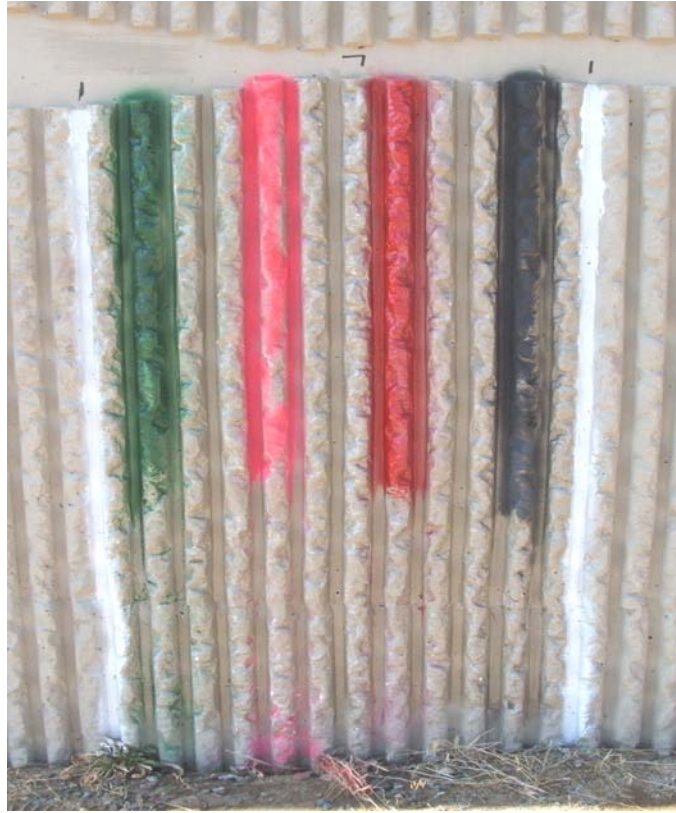
FIGURE 4.7C Removal - Fractured Fin Facing Panel 7
