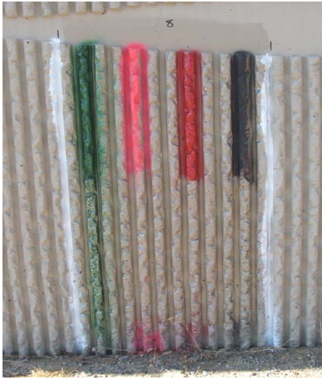
FIGURE 4.8C Removal - Fractured Fin Facing Panel 8
