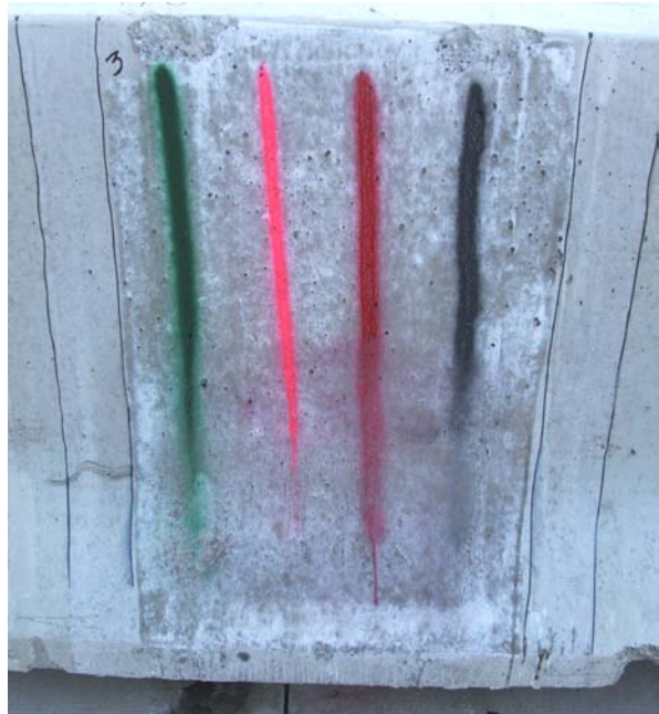
FIGURE 4.3B Removal – Unpainted Panel 3
