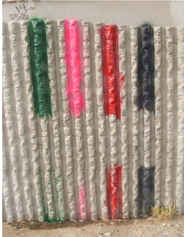
FIGURE 4.14C Removal - Fractured Fin Facing Panel 14
