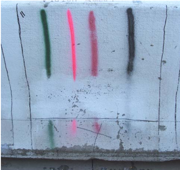
FIGURE 4.11A Removal – Painted Panel 11
