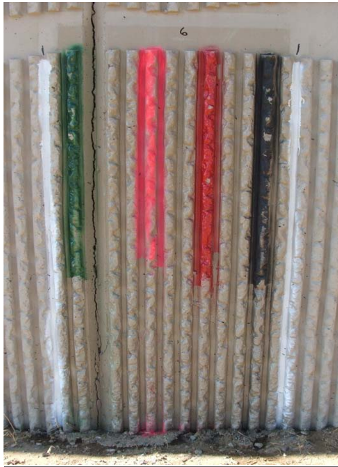
FIGURE 4.6C Removal - Fractured Fin Facing Panel 6
