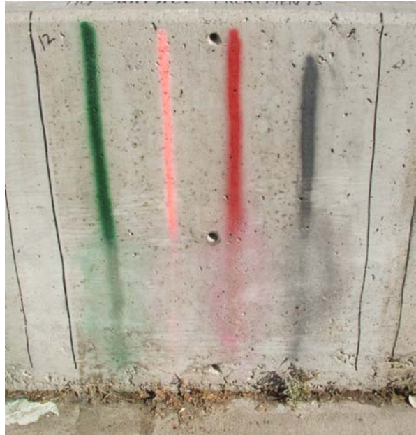
FIGURE 4.12B Removal – Unpainted Panel 12
