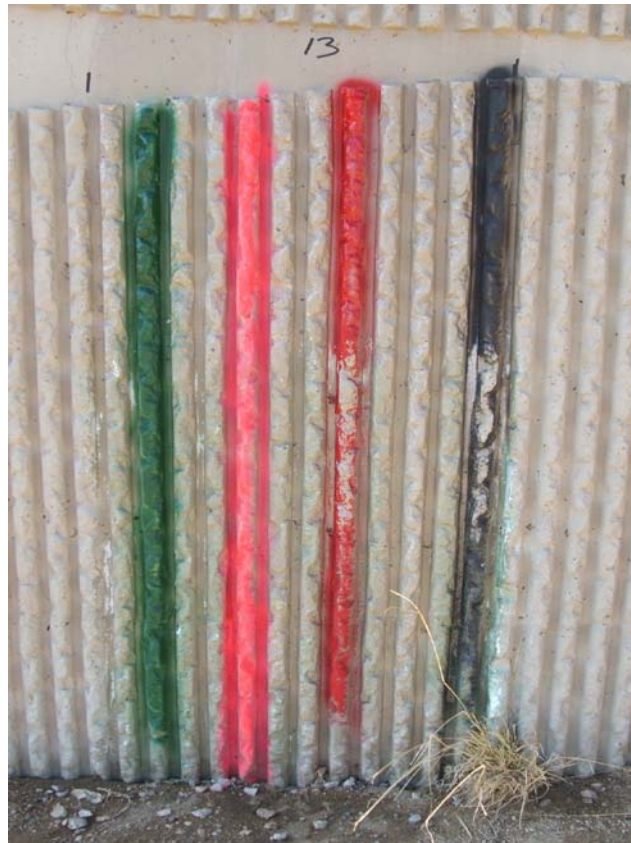
FIGURE 4.13C Removal - Fractured Fin Facing Panel 13
