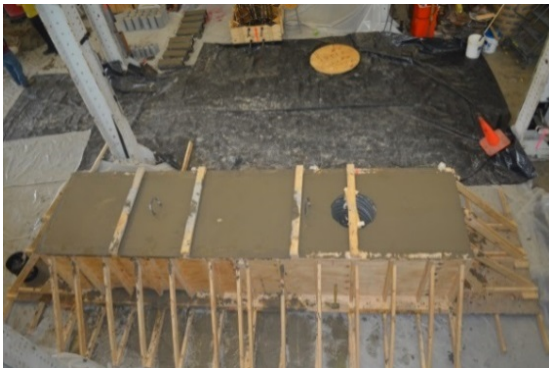
(g) Finished Surface
