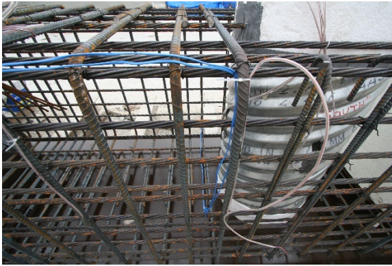
(a) PSV-28A Strain Gauged Mild Steel Reinforcement and Corrugated Steel Pipe
