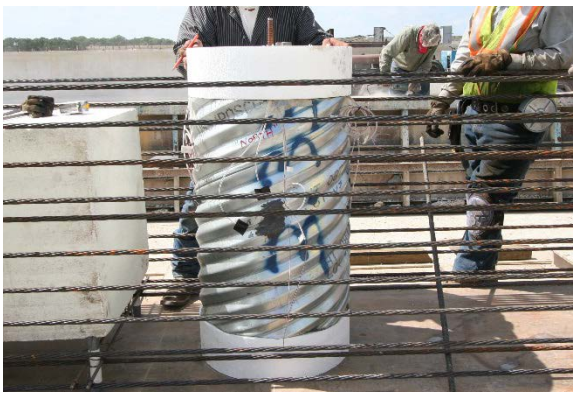
(c) PSV-28A Corrugated Pipe Secured to Prestressing Bed
