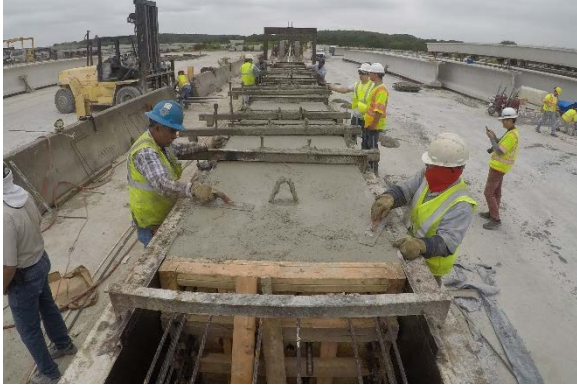
(a) Trowel Finishing
