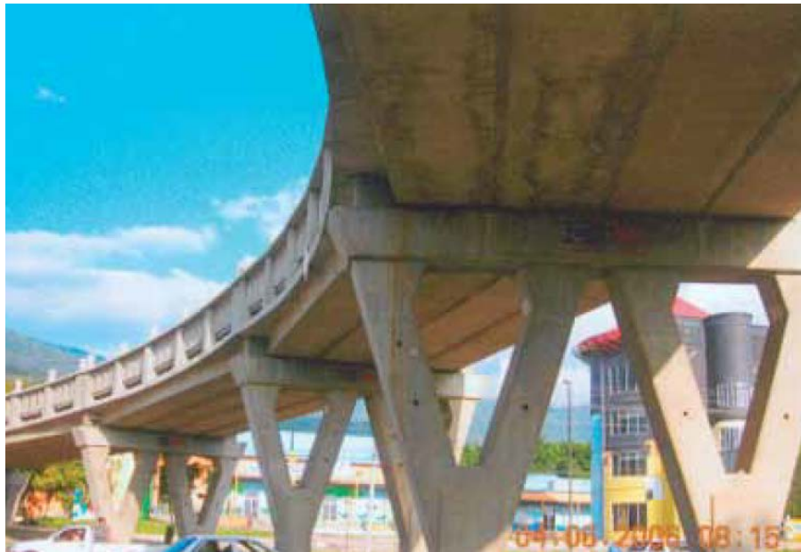
(b) The Underside of the Completed Bridge in Honduras
