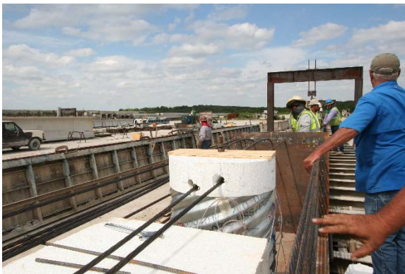
(a) Strands Placed Through PSV-28A Forming Plug
