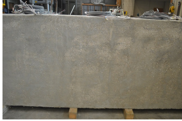
(b) Span - Repairs
