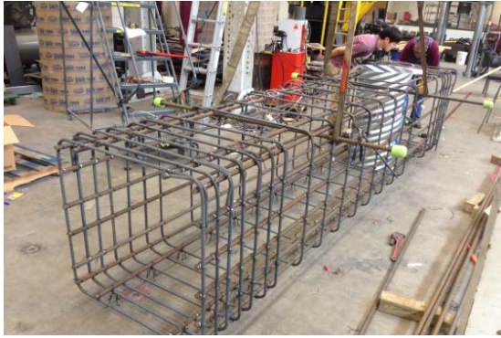
(a) Steel Reinforcement Cage
