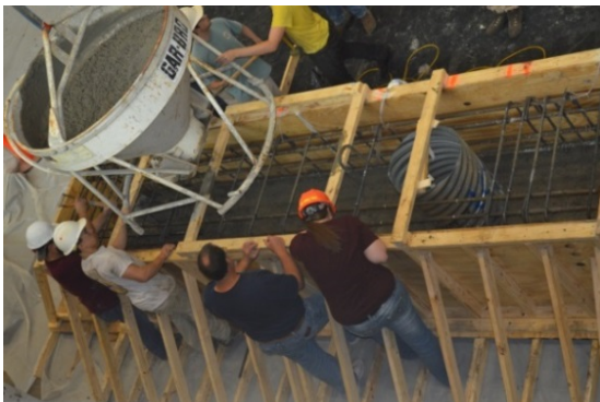
(e) Corrugated Steel Pipe Anchorage
