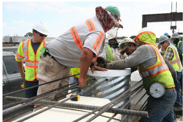
(b) Workers Feeding Strands Through PSV-28B Corrugated Steel Pipe
