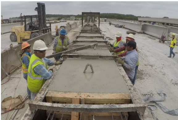
(c) Removing All-Thread Rods Securing Polystyrene Voids
