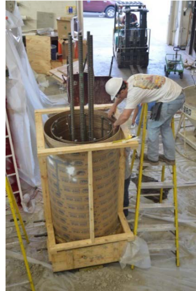
(b) Octagonal Base Formwork and Sonotube Attachment
