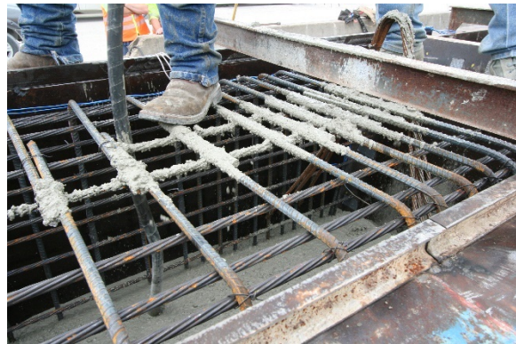
(b) Concrete Consolidation
