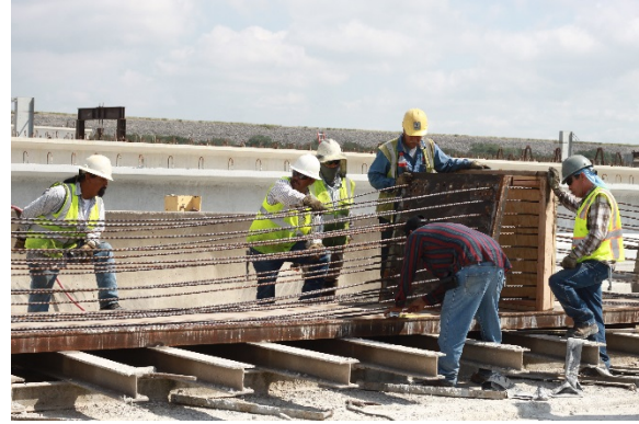
b) Prior to Stressing Initial Group of Strands
