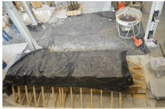
(h) Impermeable Curing Tarp
