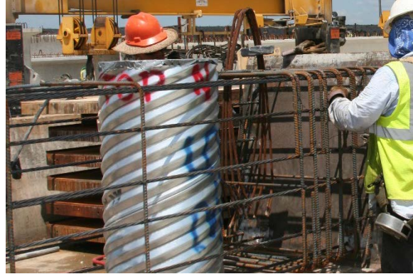
(b) Top of Phase 1 Corrugated Steel Pipes (Typ.)
