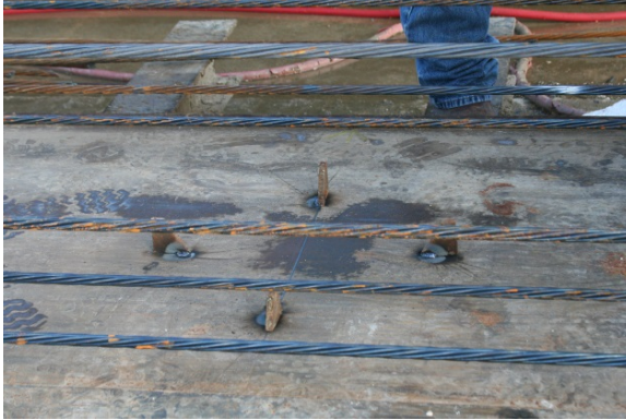
(a) Phase 1 Welded Metal Tabs Securing Corrugated Pipes (Typ.)
