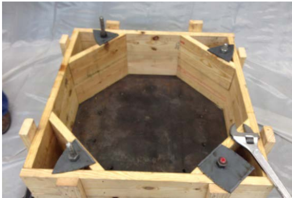
(a) Column Base Formwork Installation
