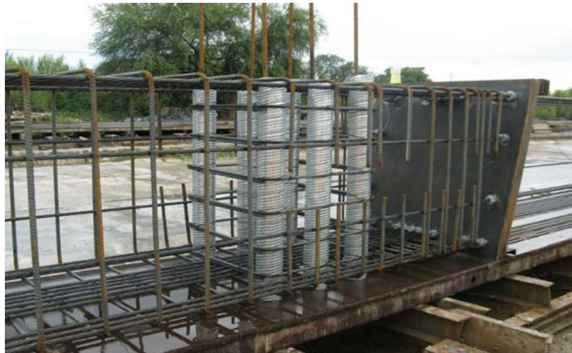
Figure 2.16. Pretensioned Precast Cap (Miller et al. 2014).
