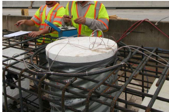
(b) Hoops at Top of Steel Pipe
