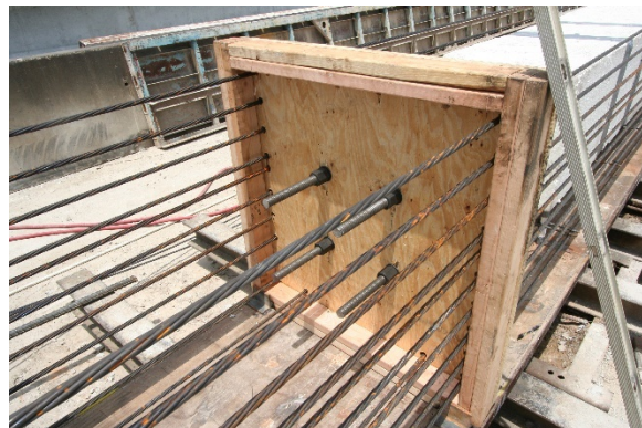
(b) Phase 2 Actuator Load Assembly Installed
