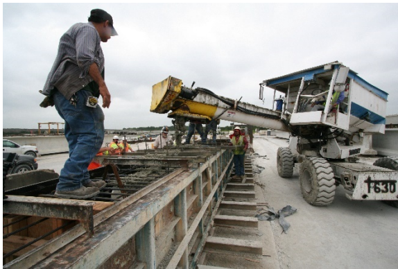
(a) Concrete Placement
