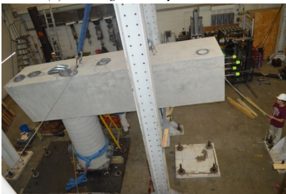
(c) Bent Cap Positioned on Column
