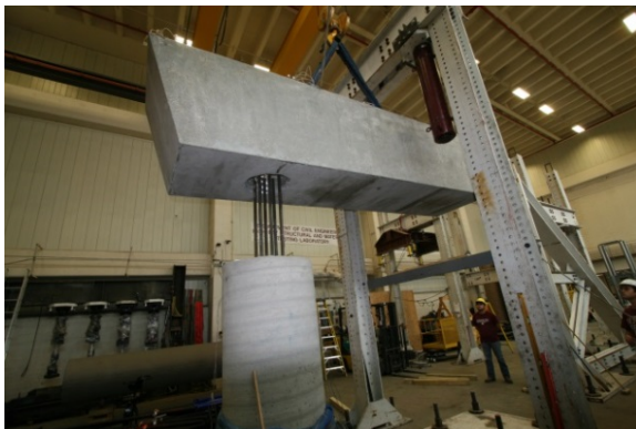
(a) Placing Bent Cap on Column
