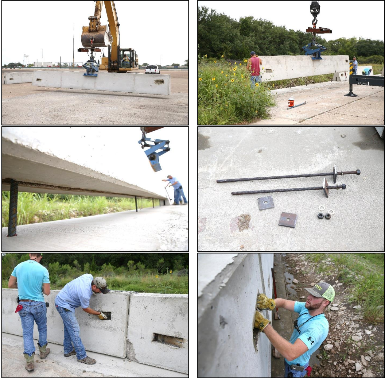
Figure 3.8. Installation of Restrained Safety-Shape Concrete Barrier on Concrete Bridge Deck.
