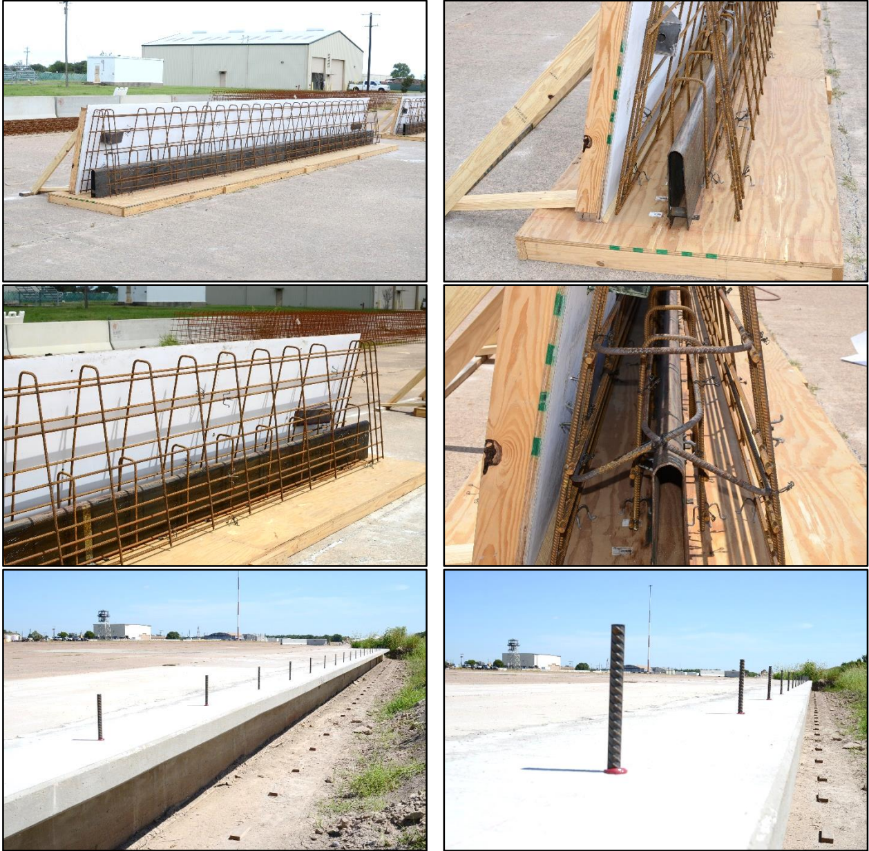
Figure 3.7. Restrained Safety-Shape Concrete Barrier under Construction.
