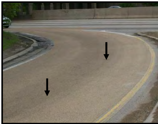
HFS Install Condition 09/2007
