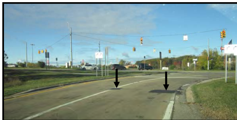
Maintenance Patching on HFS
