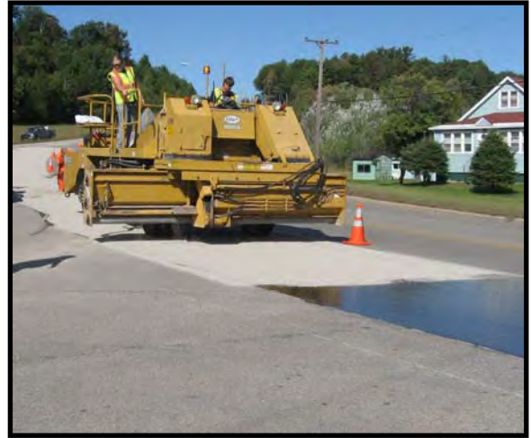
Figure 4: Spreading Aggregate Over Epoxy Resin
