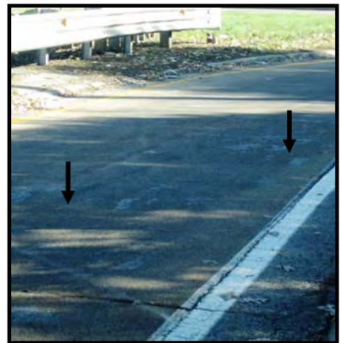
Current Condition of the HFS
