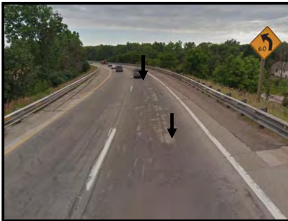
Surface Condition July 2011
