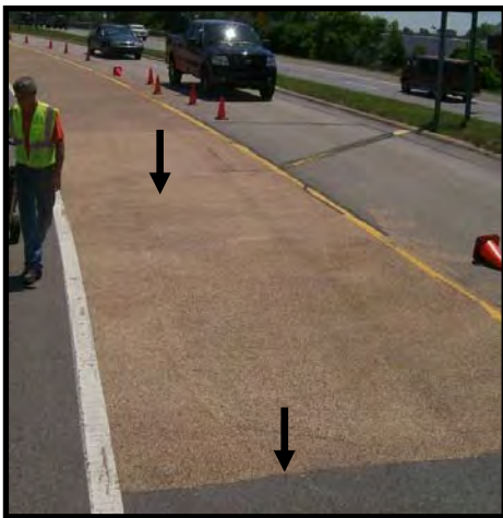
HFS Install Condition 09/2008
