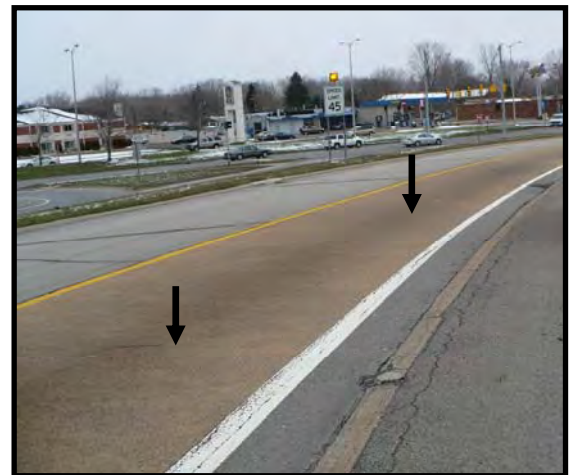
HFS Install Condition 10/2008
