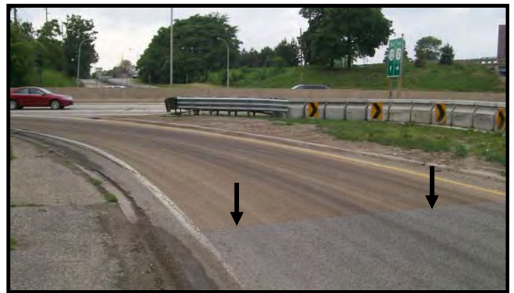
HFS Install Condition 09/2007
