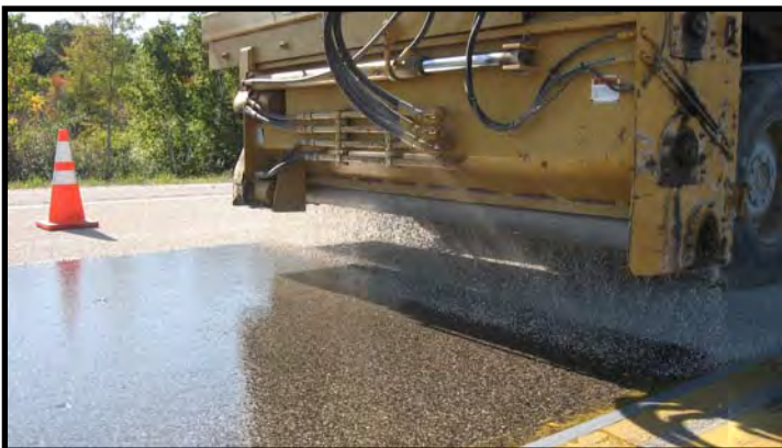
Figure 5: Spreading Aggregate
