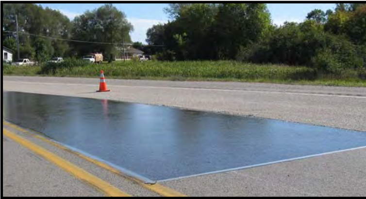
Figure 3: Epoxy Resin Applied to Pavement
