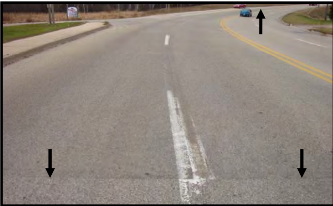
HFS Current Condition
