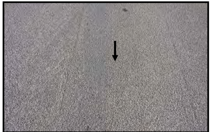
HFS Install Condition 09/2009
