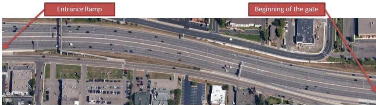
Figure 4.8 Test Site on I-394 in relation to the upstream entrance ramp.
