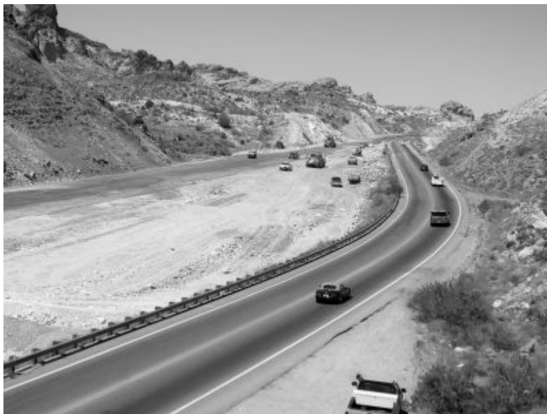
Figure 2 – Construction Along the Steep Grade on State Route 68
