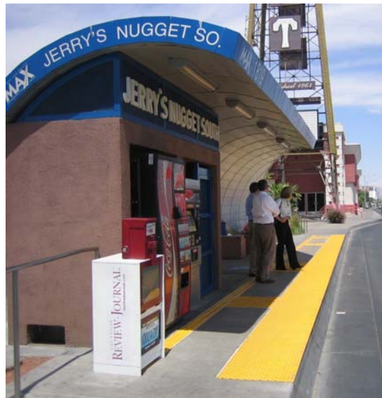
Figure 2-3: Typical MAX station (Jerry's Nugget South)
