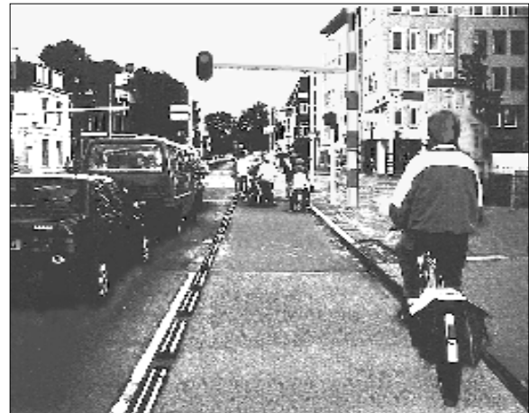
Bicycle lane in Frankfurt, Germany separated from motor vehicle traffic by a series of rubberized curbs, anchor bolted into the street pavement.
