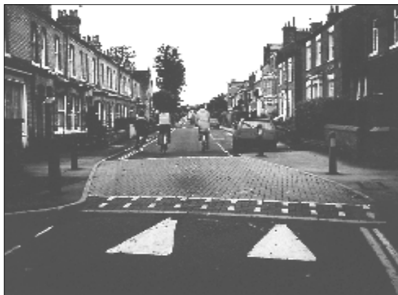
Speed table used to slow vehicular traffic on a residential street in York, England.
