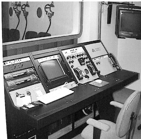
(Control Console with manual and computer controls)
