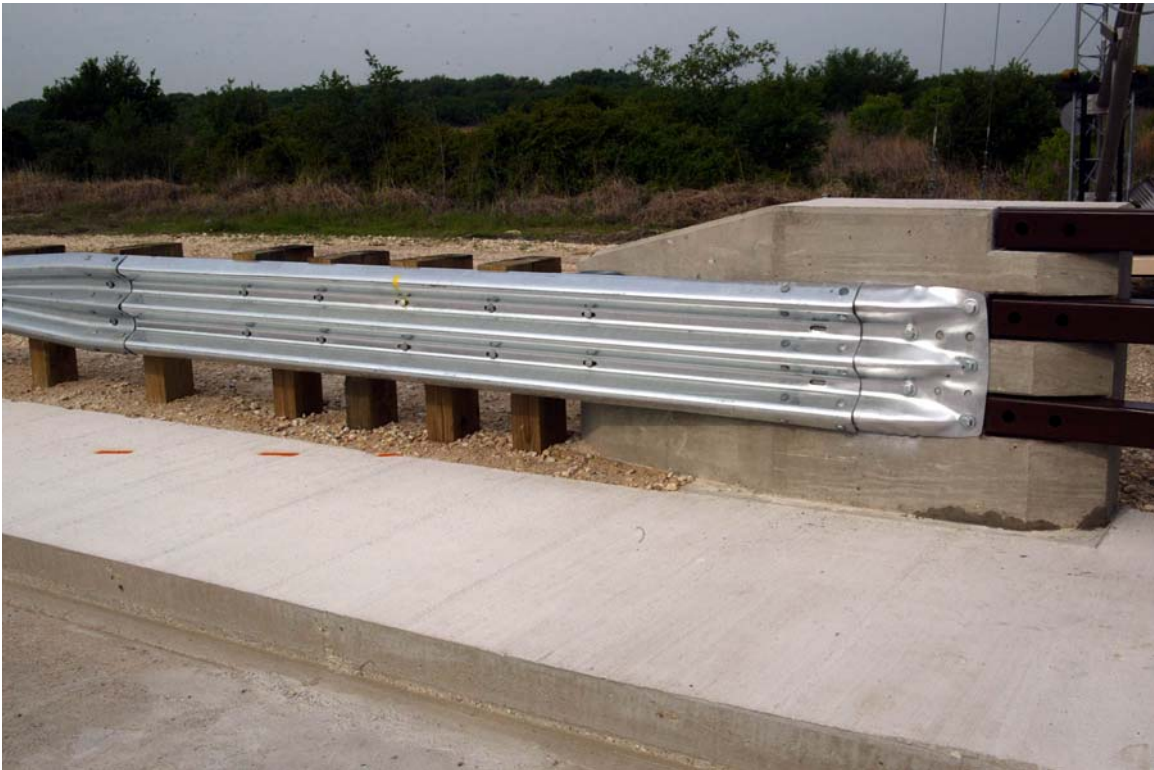
Massachusetts Transition to Concrete Wall
