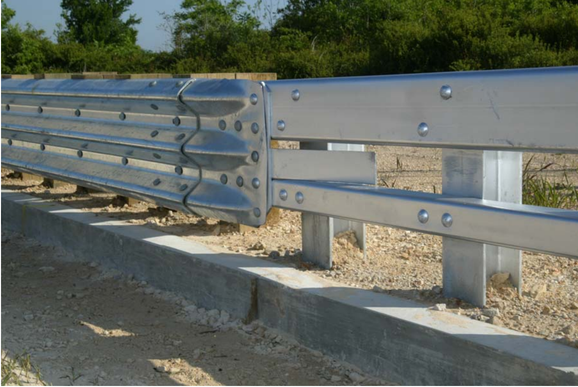
New Hampshire Transition to Two-Bar Bridge Rail
