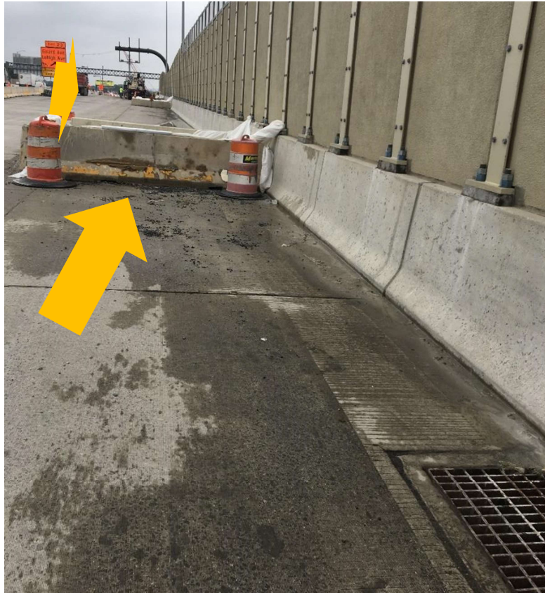
Figure 6-13: Inlet draining to SMP D, with construction blockade immediately upstream shown by the big yellow arrow. The smaller arrow is pointing to the construction blockade recently installed next to the inlet to SMP G.
