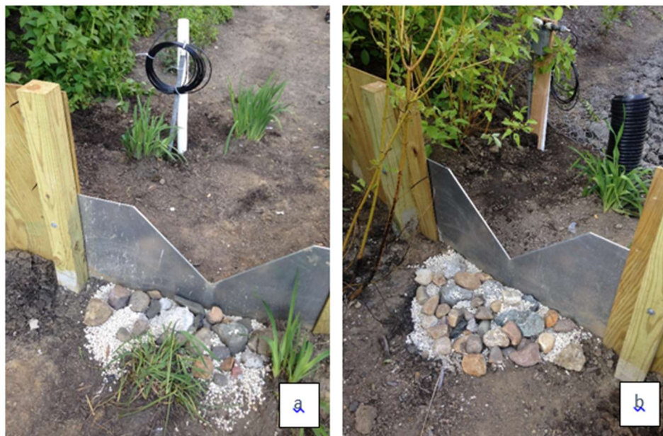
Figure A2-3: (a) Upstream and (b) Downstream V-Notch Weirs
