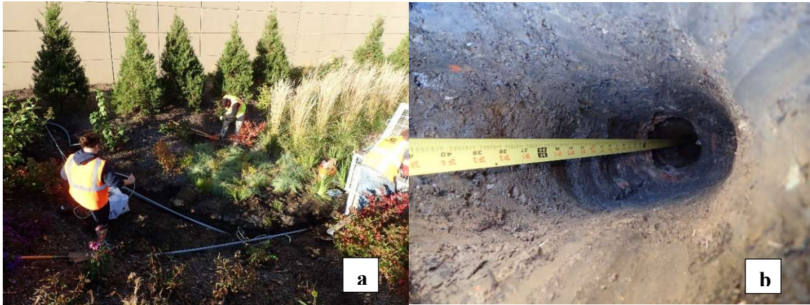
Figure 3-15: Digging and Laying Conduit in SMP D (a). Hole prior to soil moisture probe installation (b)
