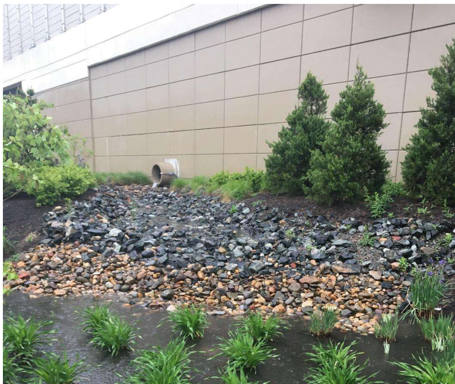
Figure 6-3: SMP C Rock Stilling Basin during May 5, 2017 Storm
