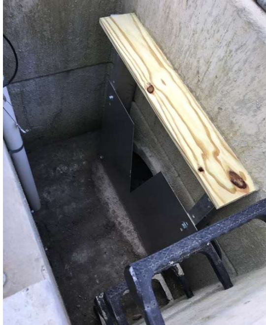
Figure 3-17: Outlet V-Notch Weir, Weir Cover, and slotted pipe for pressure transducer (top left).
