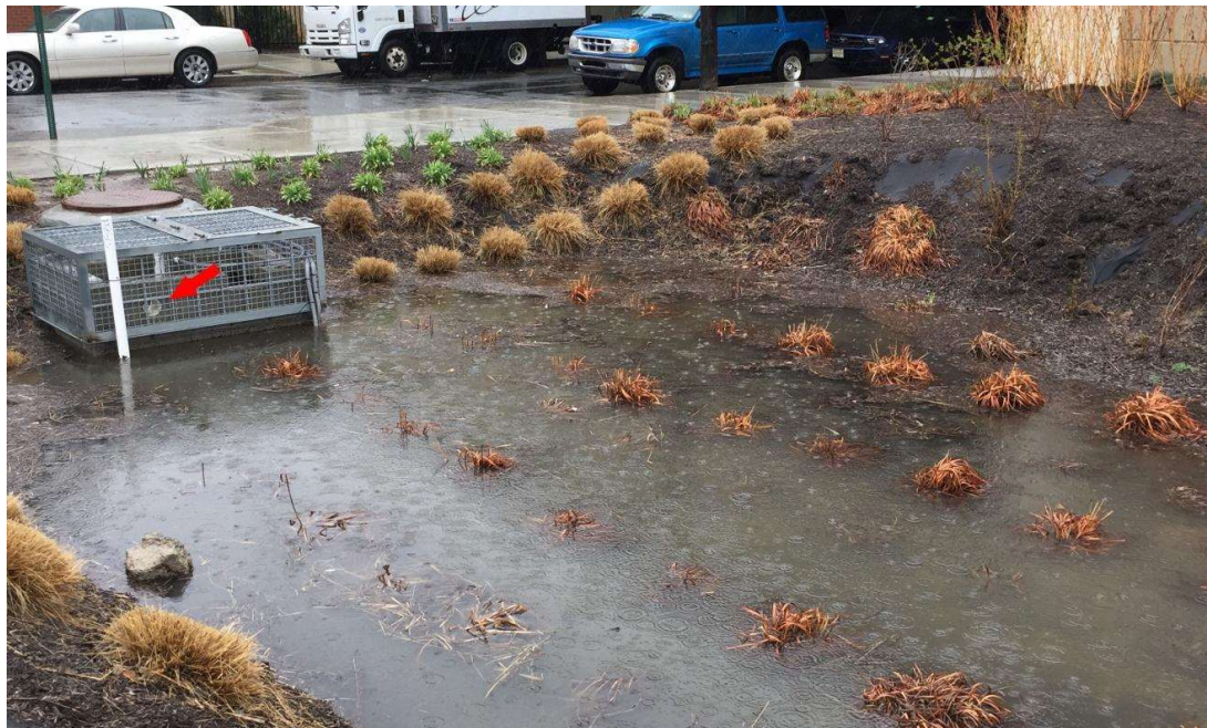
Fig. 6-22. Photo of the extent of ponding on SMP device C. This photo was taken on 31 March 2016 during a 1.54-inch rainstorm. Note that the height of ponded water is still well below the outlet drain (red arrow).
