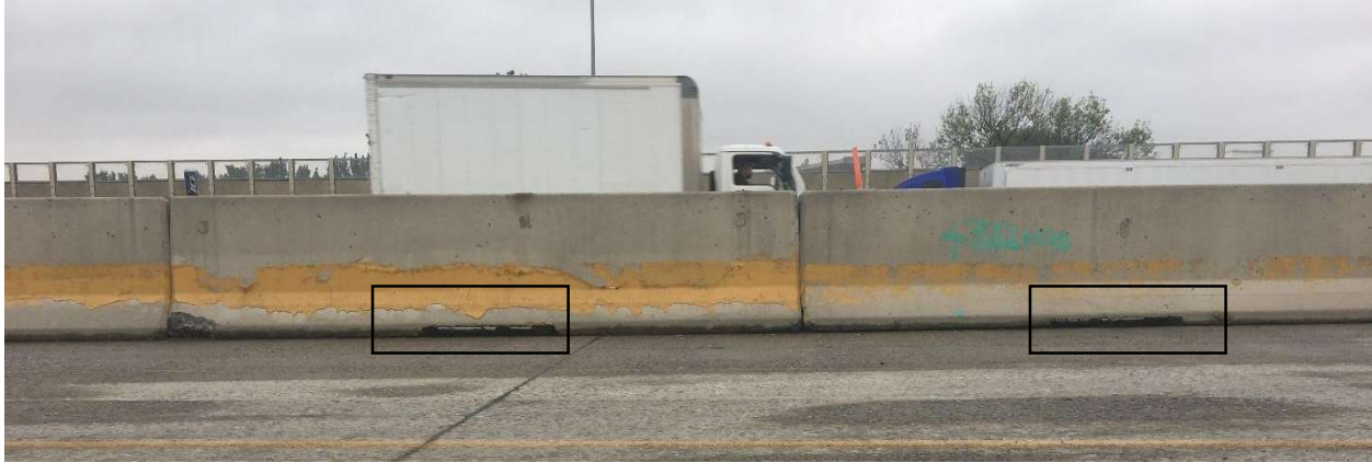
Figure 6-11: New Jersey Barriers defining the temporary travel lanes. The opening is circled to show where flow can get through.
