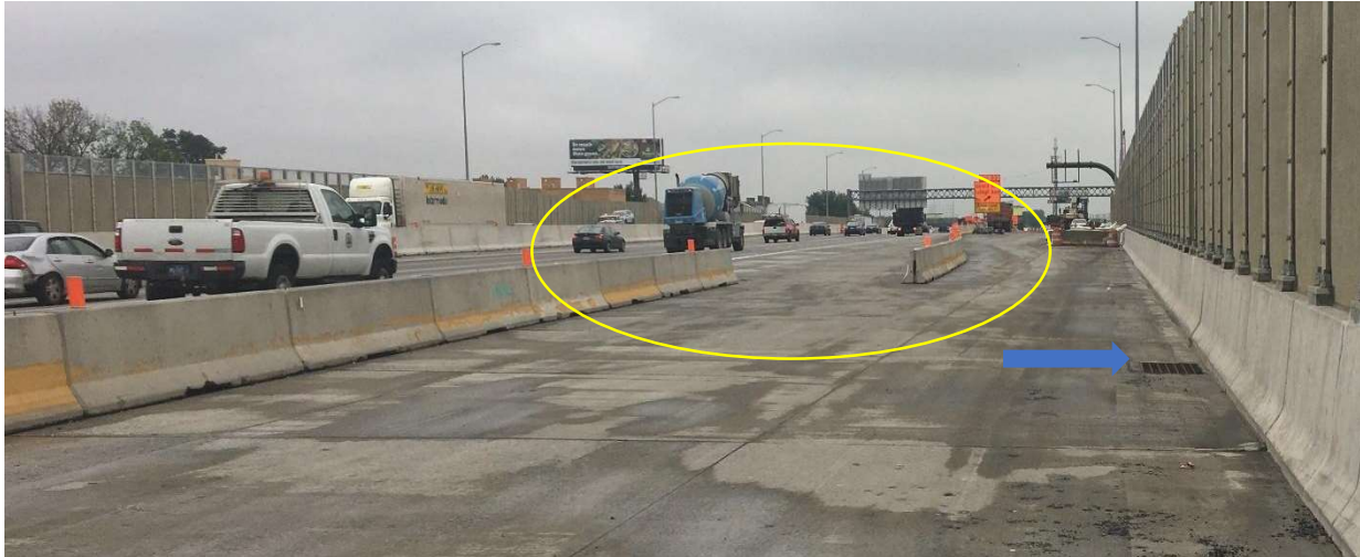
Figure 6-12: Barriers moved from single line, to form an opening in front of SMP C exit ramp inlet (shown on the right edge of photo, indicated with the blue arrow)
