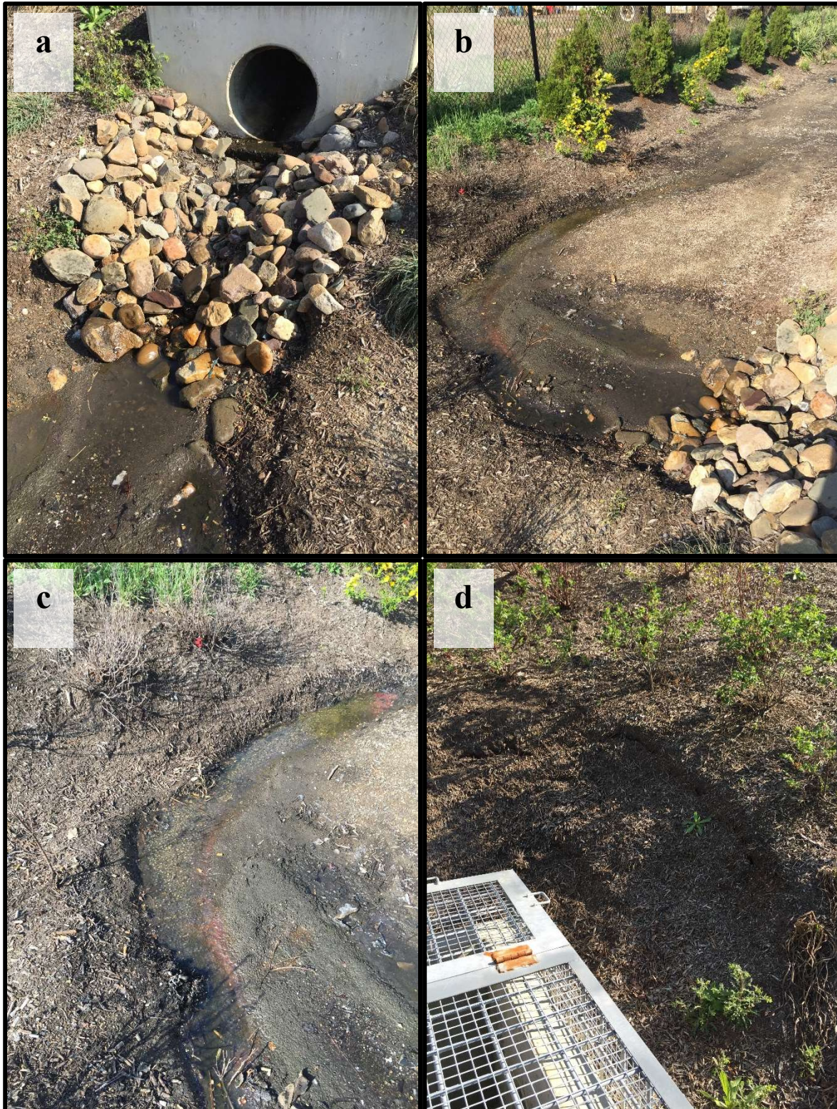
Figure 8-5. SMP H. Photos were taken 4-14-2017, a week after the last precipitation event (4-7-2017), and there is still a small amount of standing water in the SMP (a, b, c). There is also significant scour near the inlet and soil loss near the outlet (a, b, c, d).
