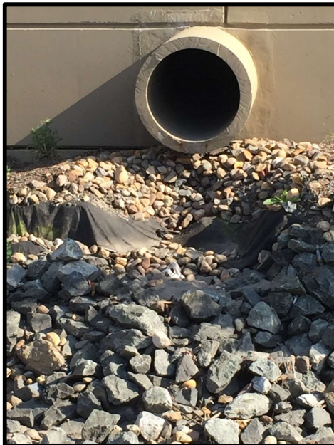
Figure 8-7. SMP J has severe erosion of the soil around the inlet and is experiencing failure of the rip rap support structure.
