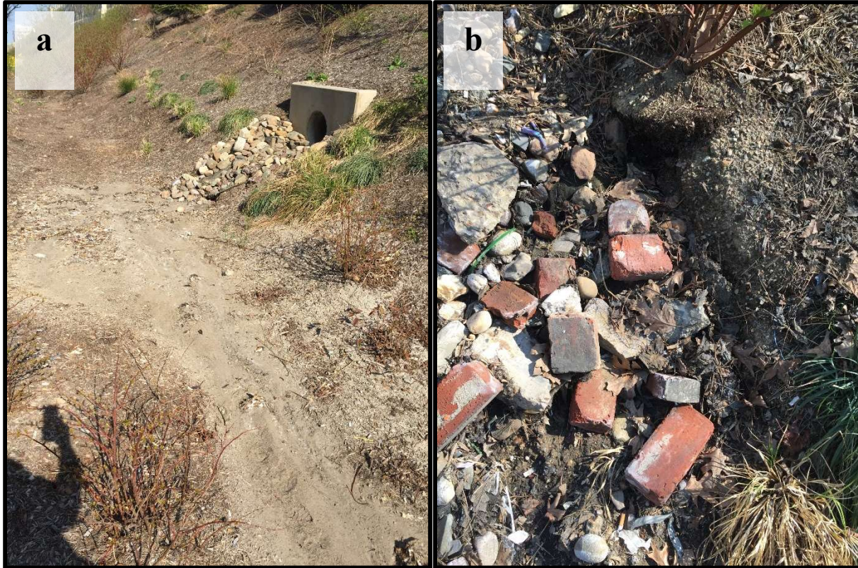
Figure 8-4. Erosion in SMP E consists of scour and soil loss at the edges of inlet rip rap (a, b). Large amounts of small trash accumulates in the rip rap (b).
