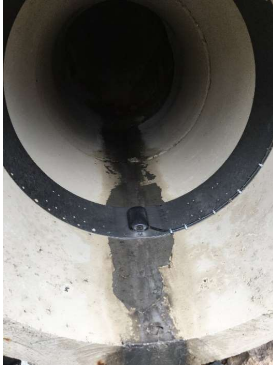
Figure 3-12: Installed Blue Siren Area Velocity Sensor
