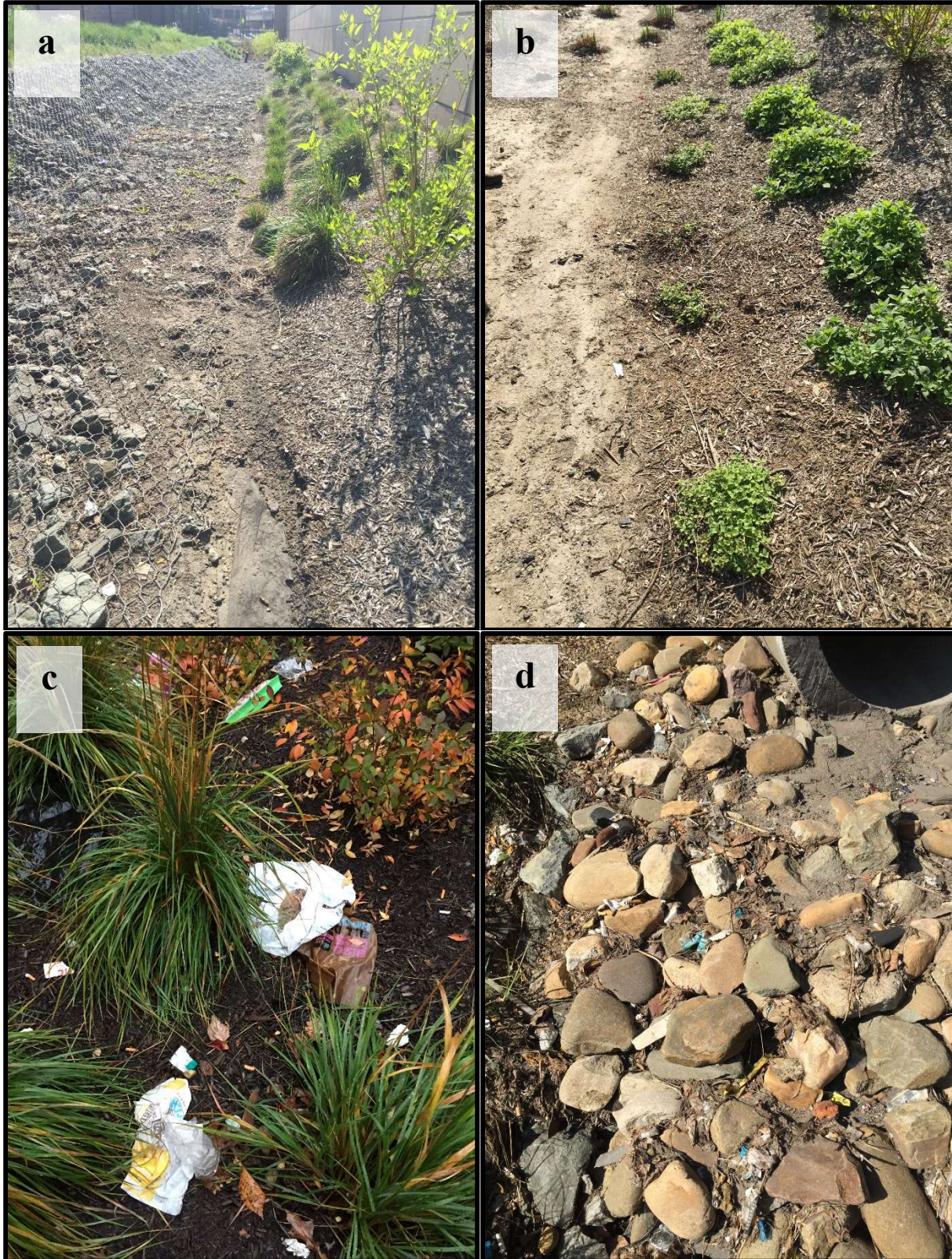
Figure 8-1. SMP A is showing signs of erosion along the lower edge of the gabion (a), along the lowest elevation of the basin (b). There is also an accumulation of large (c) and small (d) trash items.
