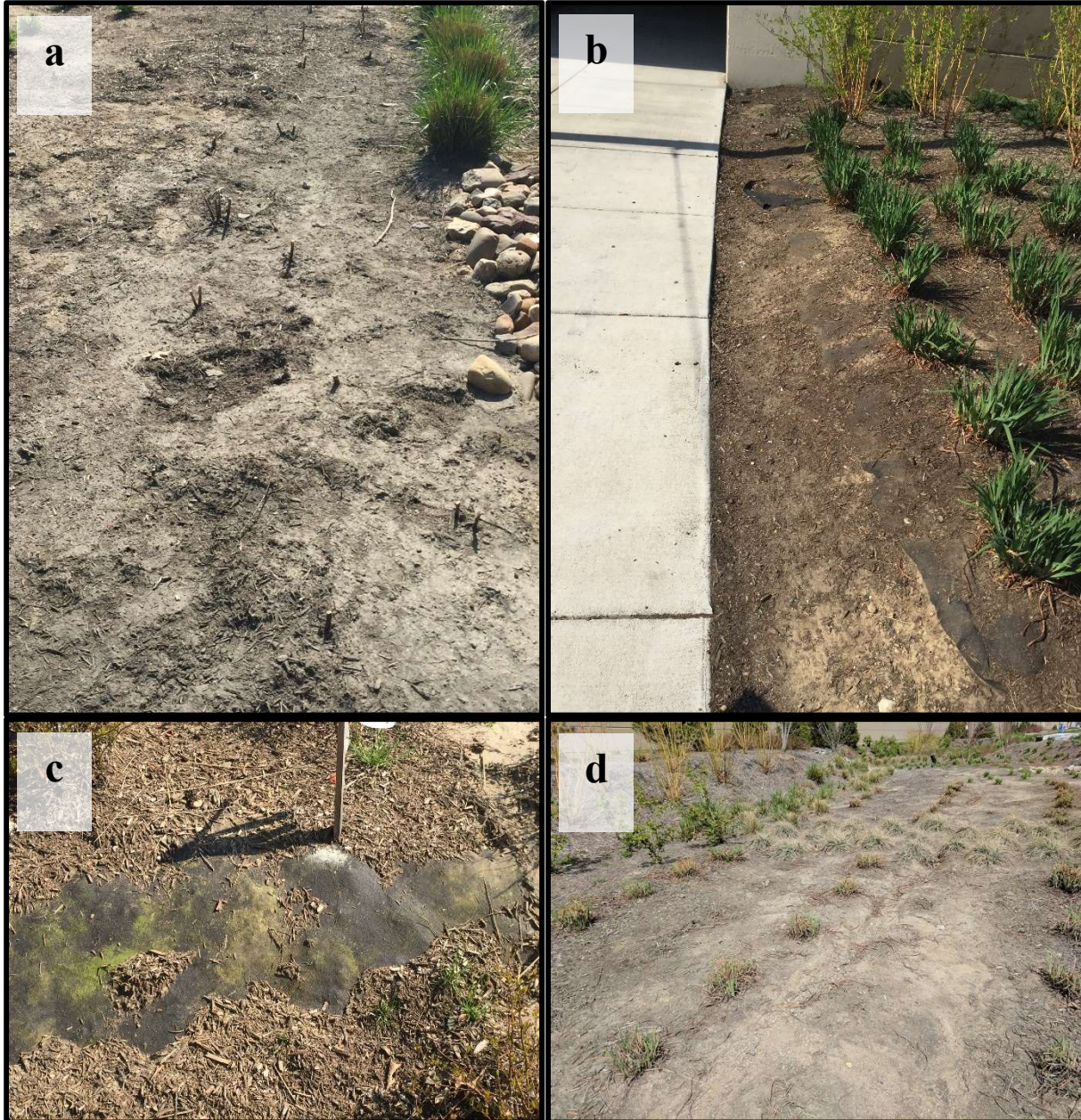
Figure 8-2. SMP C. This basin has a particularly large area and has developed signs of erosion from stream-like flow that occurs during precipitation events (a, d). This has had a scouring and slight channelizing effect. Placing plants in rows parallel to the flow of water may exacerbate this process. The basin edge (b) and sloped sides of the basins (c) show significant loss of mulch.
