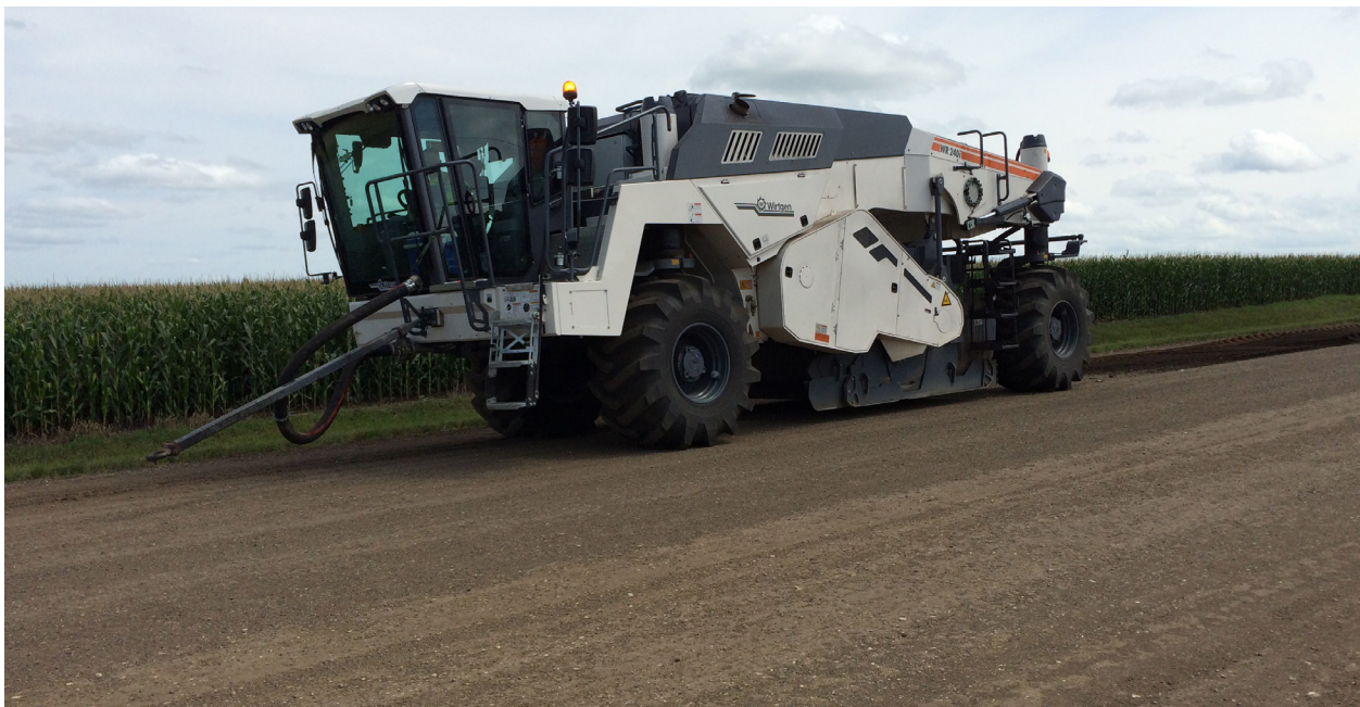
Bituminous Stabilization in Cottonwood County
