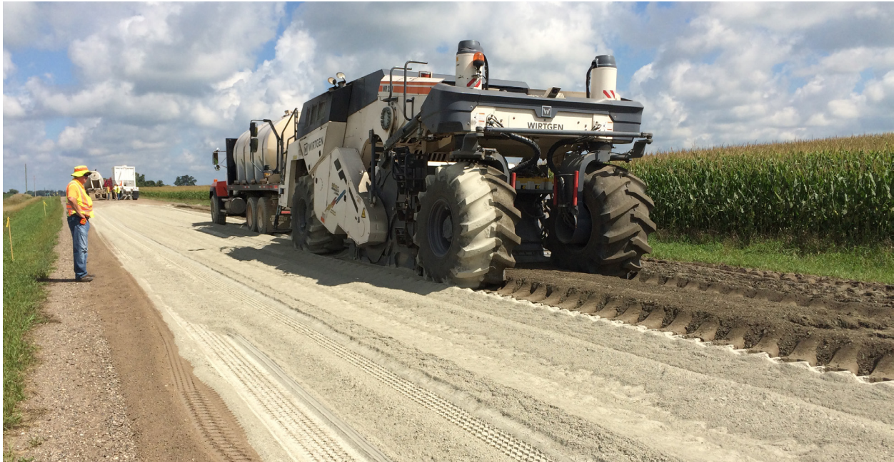
Cement stabilization in McLeod County
