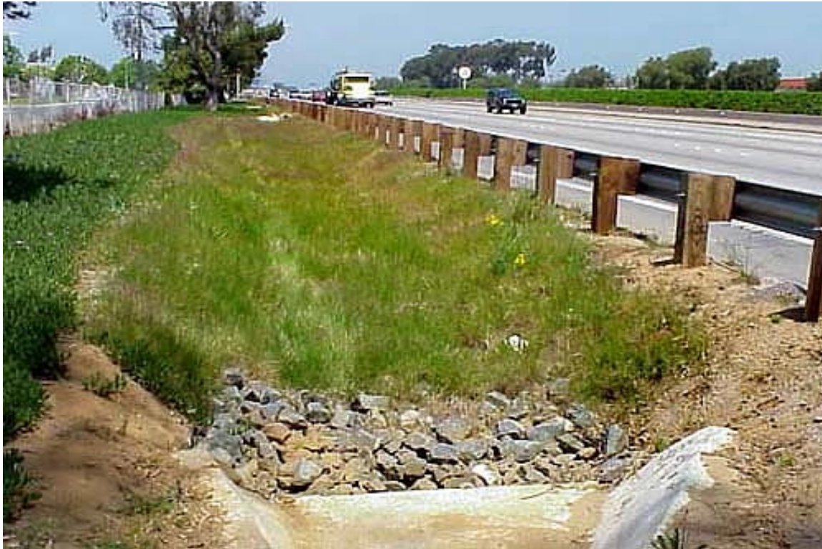
Figure 2.1 A bioswale adjacent to a highway (California Department of Transportation (Caltrans), 2015).
