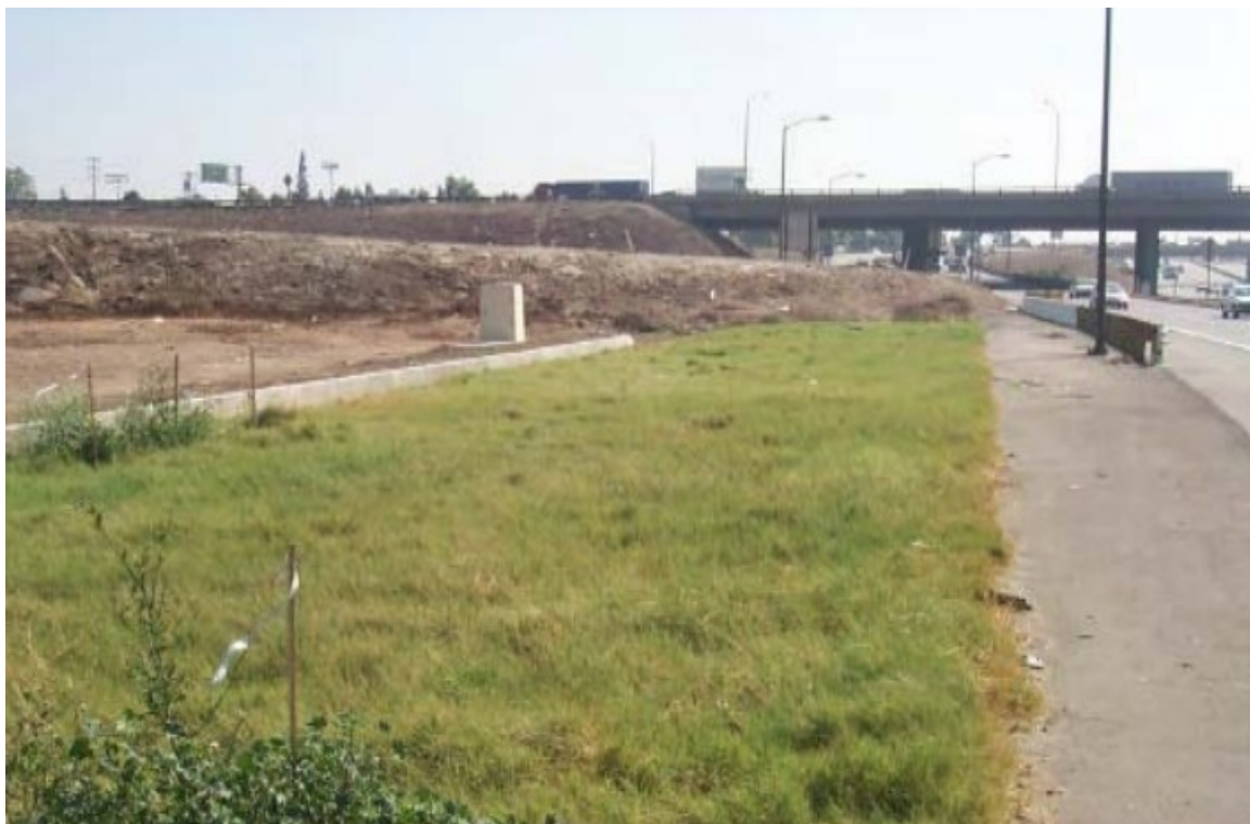
Figure 2.2 Bioslope adjacent to a highway (Caltrans, 2004).
