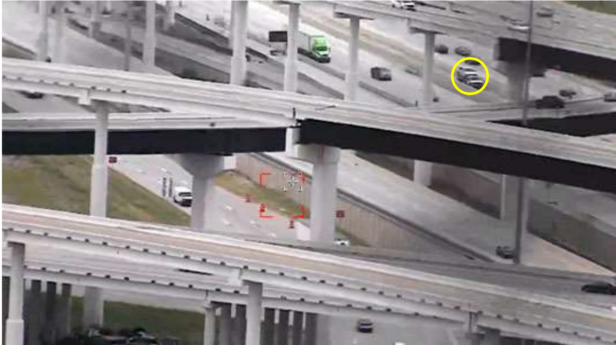
Figure 18. Example of Line of Site Obstruction from Bridges at US 290 and Beltway 8
