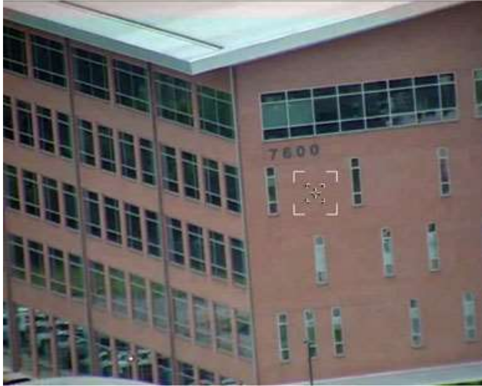
Figure 29. Images from UAS of TxDOT-Houston District Building at Maximum Zoom
