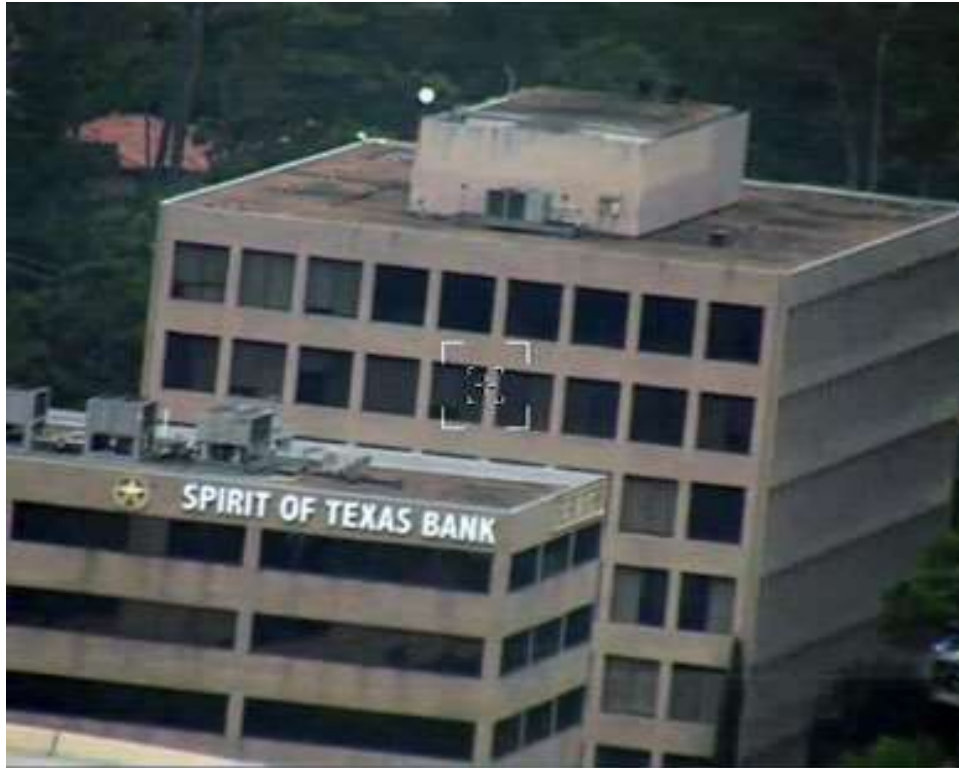
Figure 31. Images from UAS of TTI-Houston Office Building at Maximum Zoom
