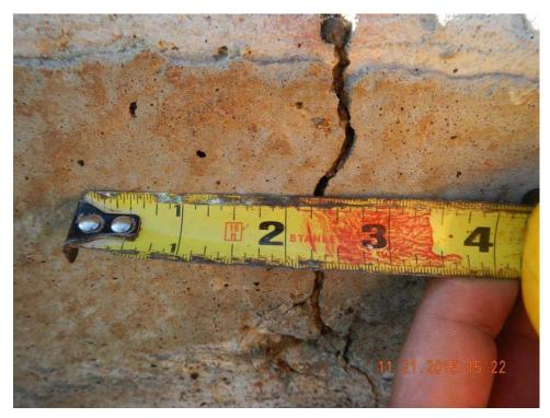
Figure 4.24 Crack width at Joint on FM 2253
