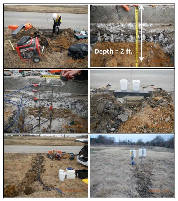
Figure 4.5 Gage installation procedures and data logger installation on SH 288
