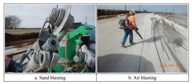
Figure 2.7 Sand blasting and air blasting
