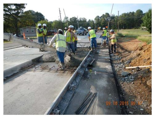
Figure 4.15 Concrete placement on FM 2253
