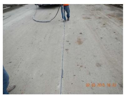
**Figure 2.9 Sealant installation**
