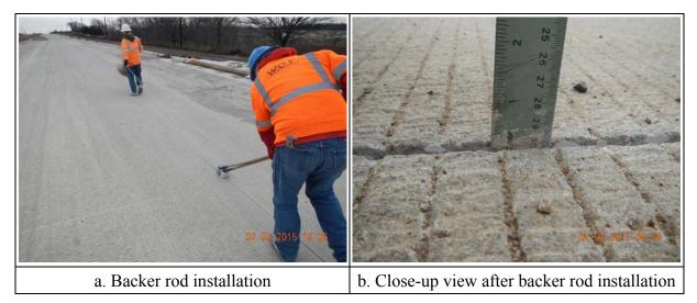
Figure 2.8 Backer rod installation
