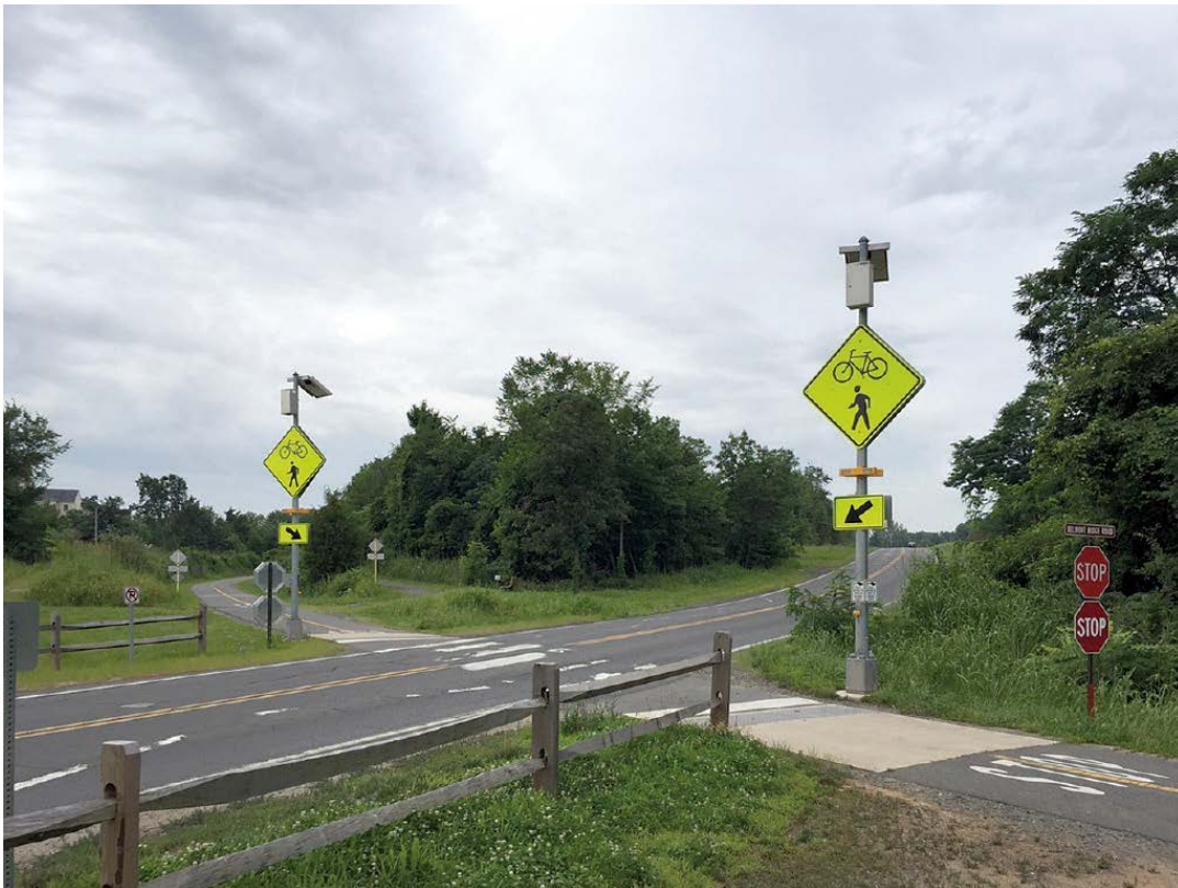
Figure 5.11: Rectangular Rapid Flash Beacon (RRFB) (N/A, N/A, N/A)
