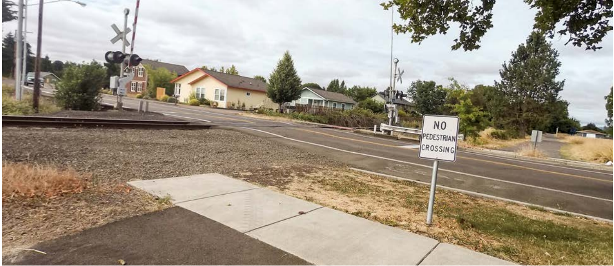
Figure 3.35: The sidewalk suddenly stops at the tracks
