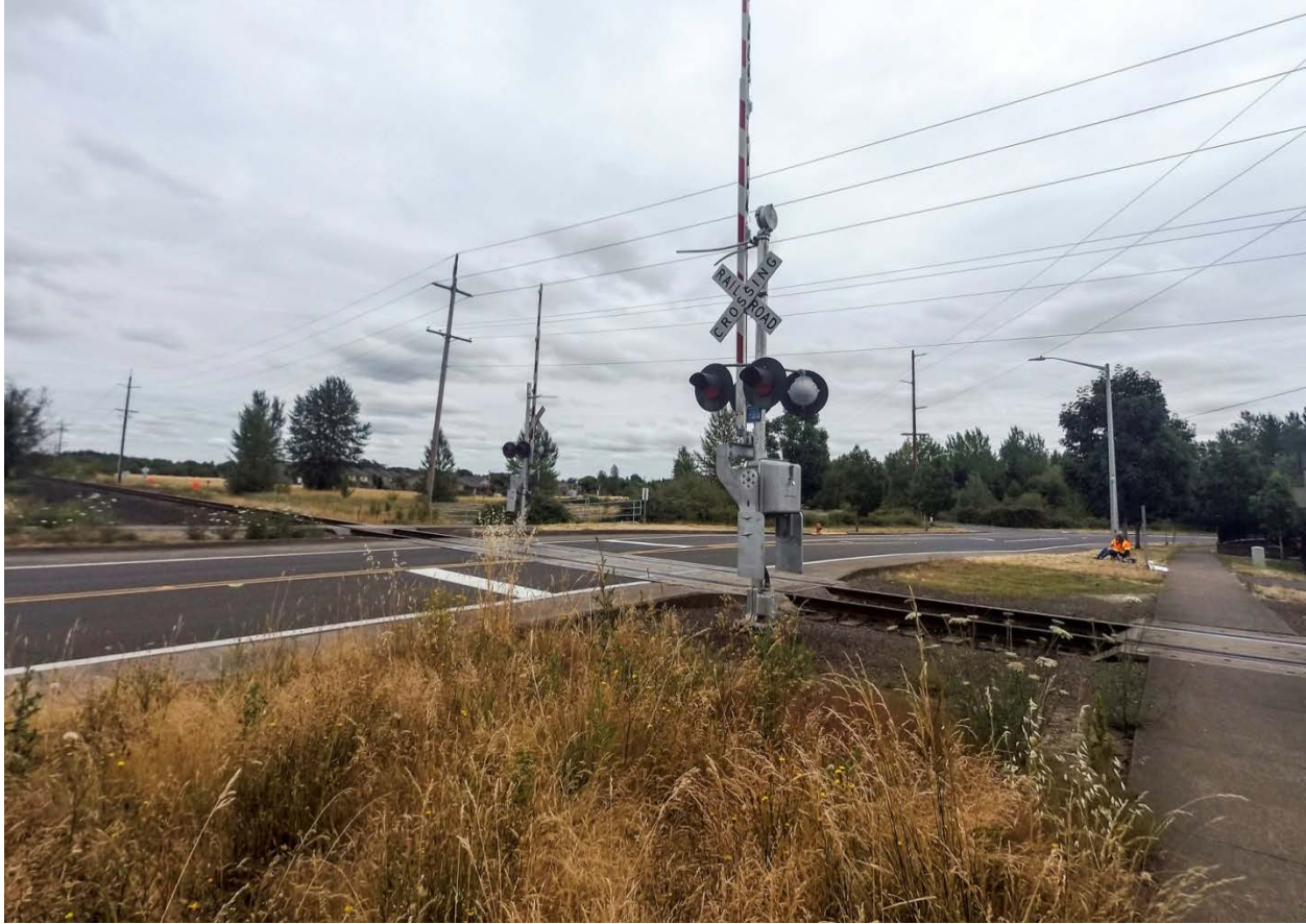
Figure 3.40: Active treatments at the NE Walnut Blvd crossing
