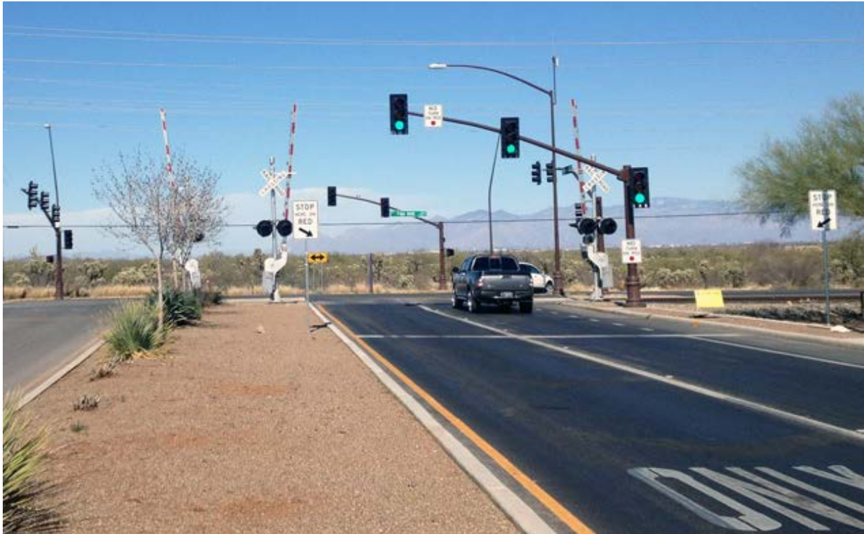
Figure 5.6: Pre-Signals/Traffic Lights (PSOMAS, N/A)
