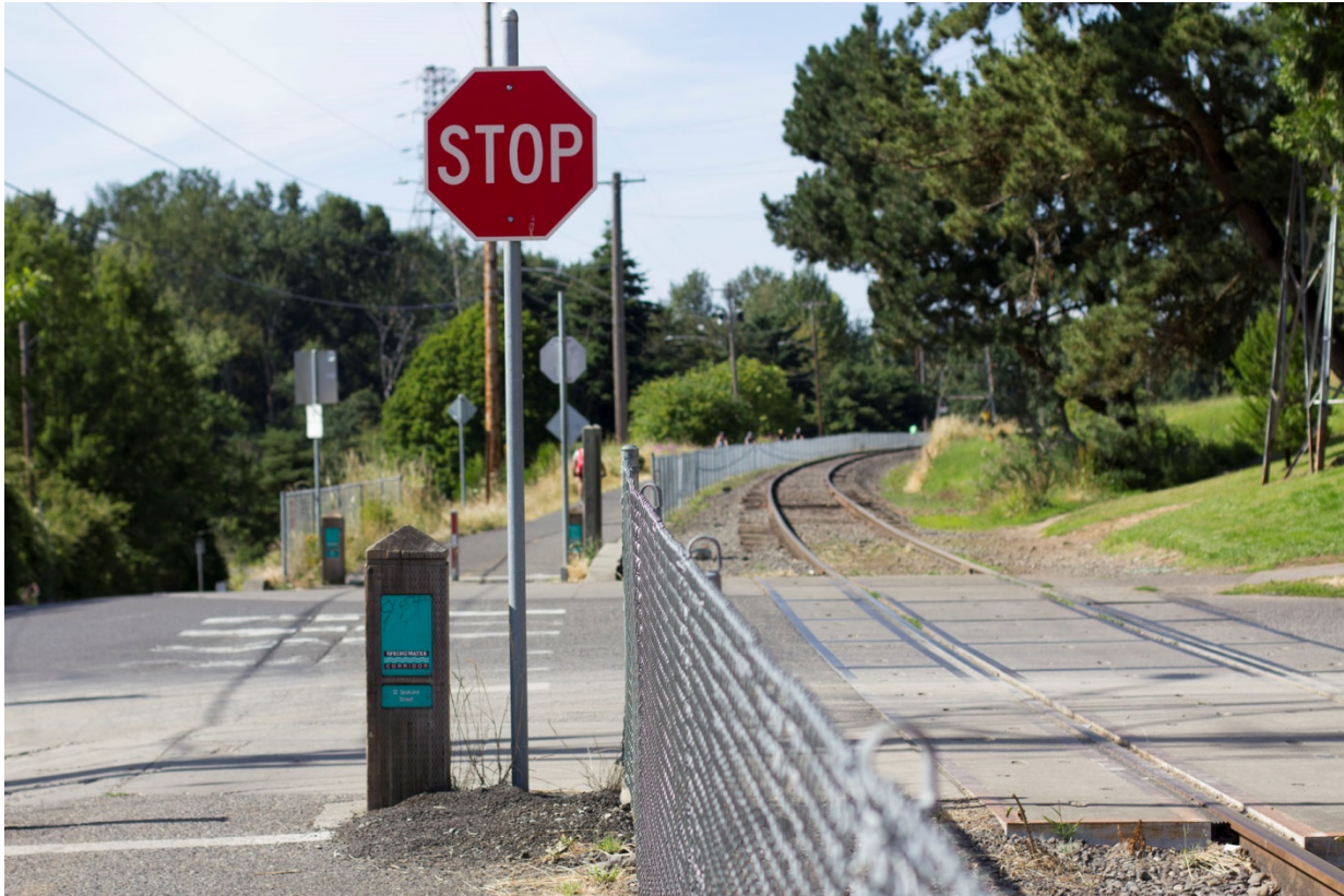
Figure 3.21: There are stop signs installed at all approaches and for all road users
