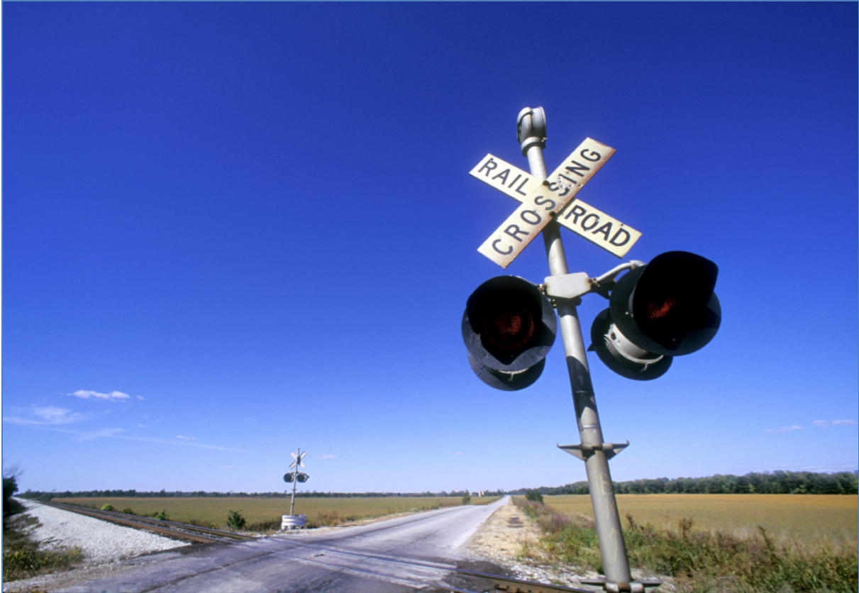
Figure 5.1: Flashing Light Signal (Mixon, 2015)
