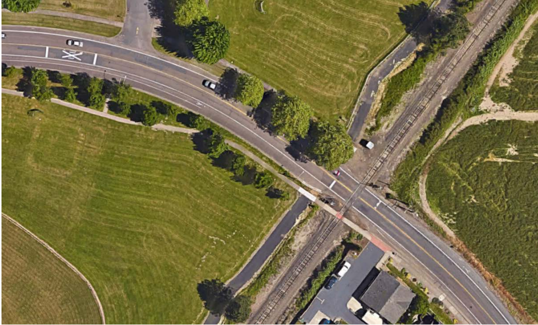
Figure 3.32: Satellite photo of the NE Conifer Blvd crossing in Corvallis, OR (Google, 2016) (Trail is marked in orange)
