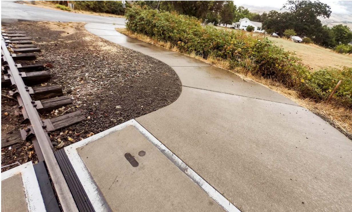
Figure 3.47: Curving the foot path enables pedestrians and bikes to cross at a 90° angle, to meet ADA access and encourages pedestrians to look to the sides before crossing
