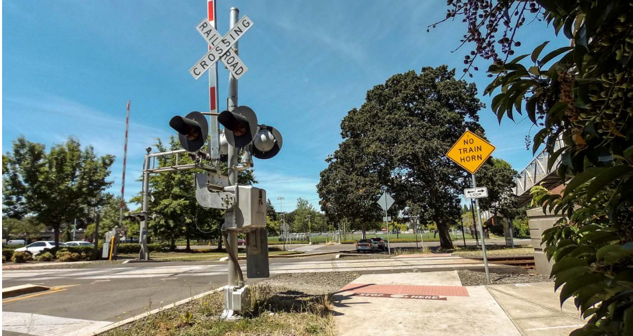
Figure 3.27: Active and passive treatments at the SE Mill St Crossing
