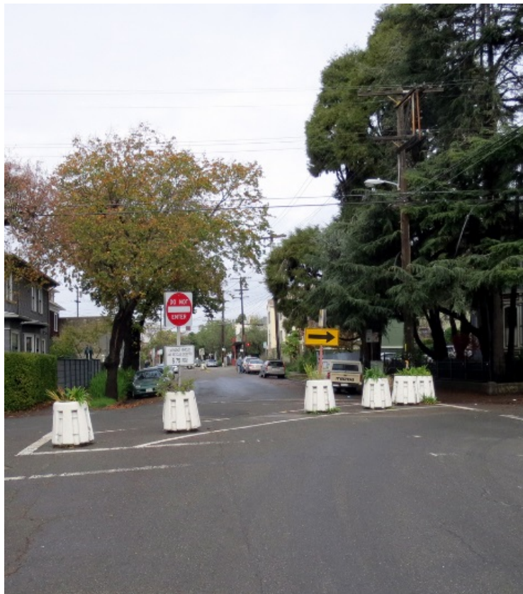
Figure 5.29: Bollards used to keep vehicles from entering, (N/A, N/A)
