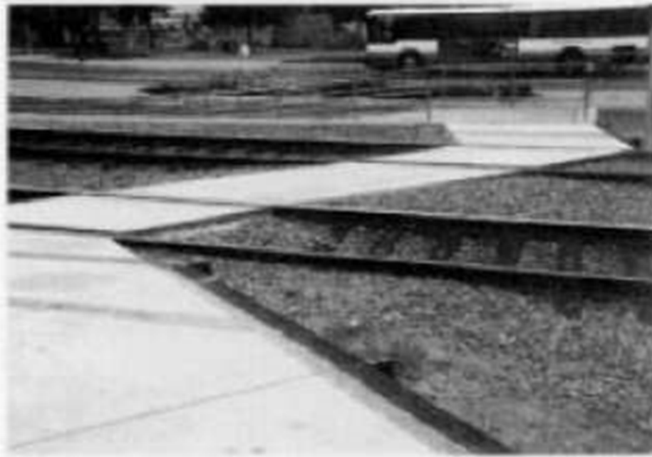
Figure 5.33: Channelization, (Korve, Hans W. , Jose I. Farran, Douglas M. Mansel, et al., 1996)
