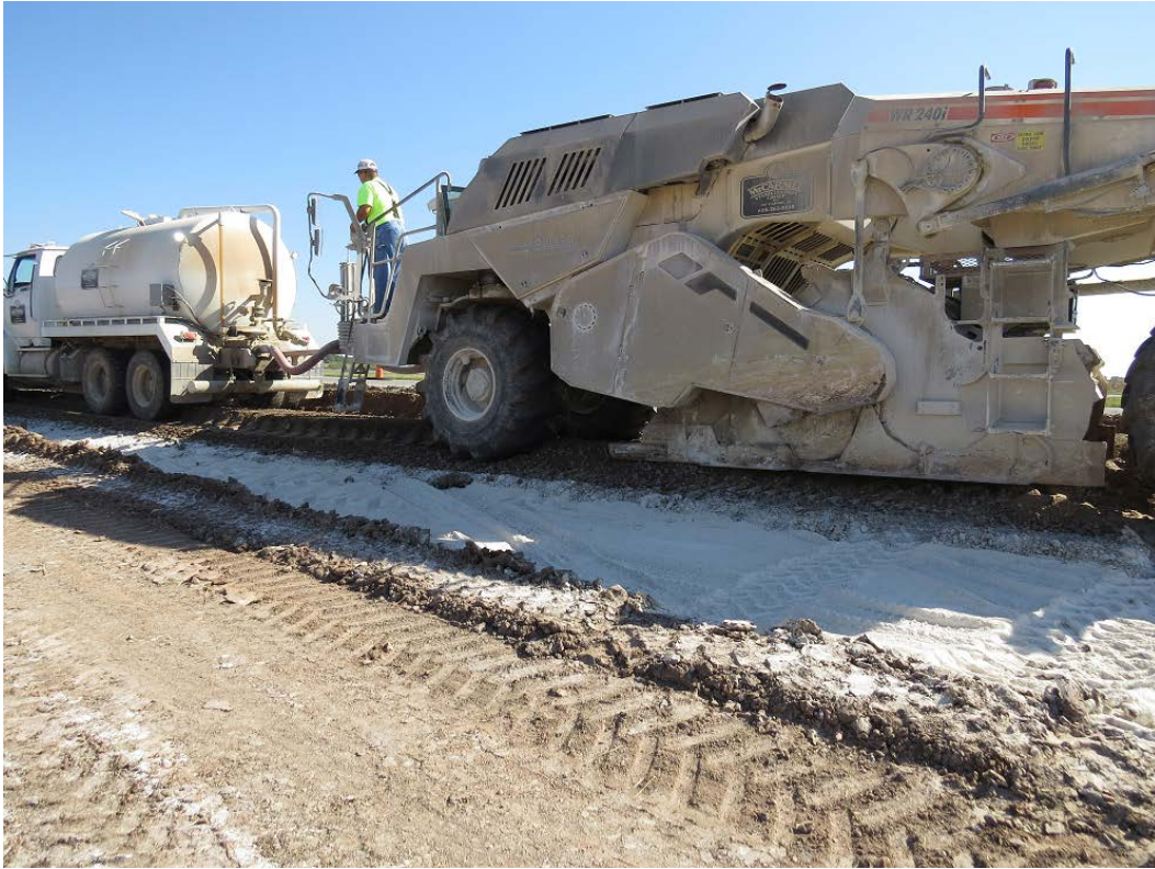
Figure 5.2: The Rotary Mixer and the Attached Water Tank
