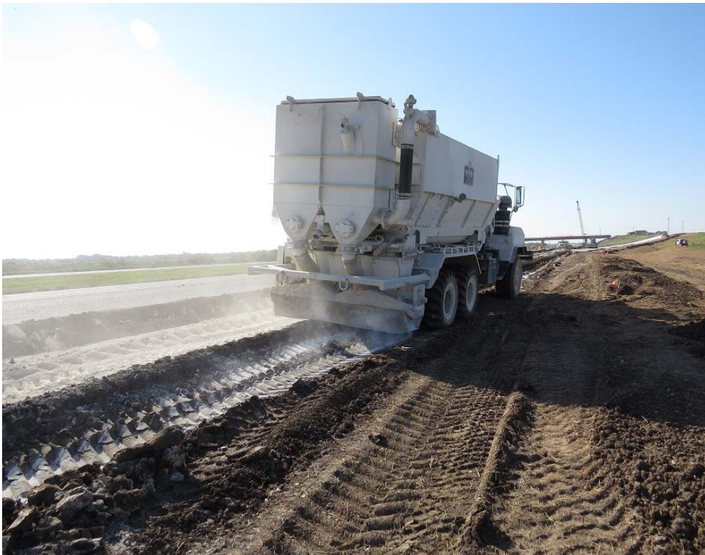
Figure 5.1: A Spreader Truck Distributing LKD
