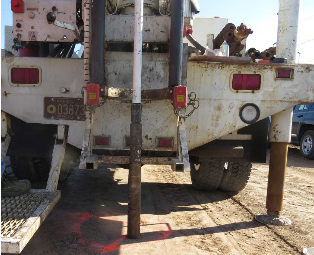
Figure 5.7: Taking Shelby Tube Soil Samples (KDOT Drill Rig)
