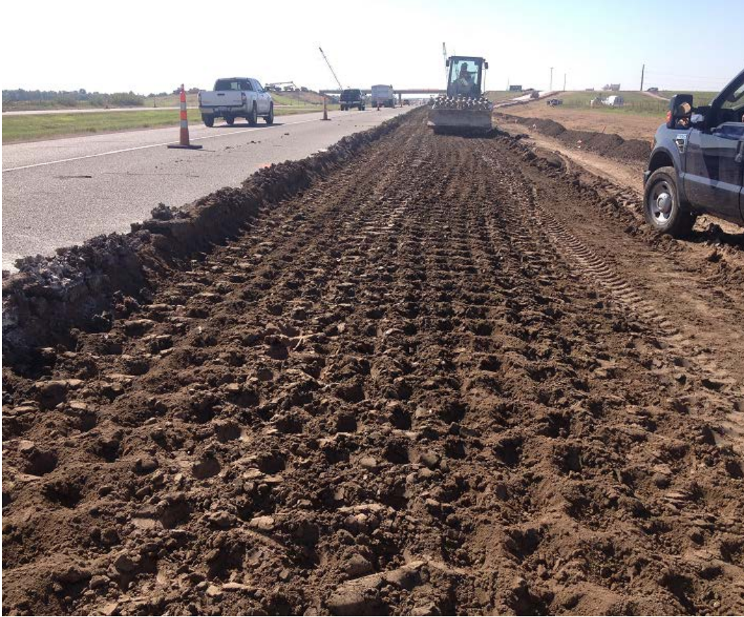
Figure 5.3: Compacting LKD-Soil Mix Using a Vibratory Pad Foot Roller
