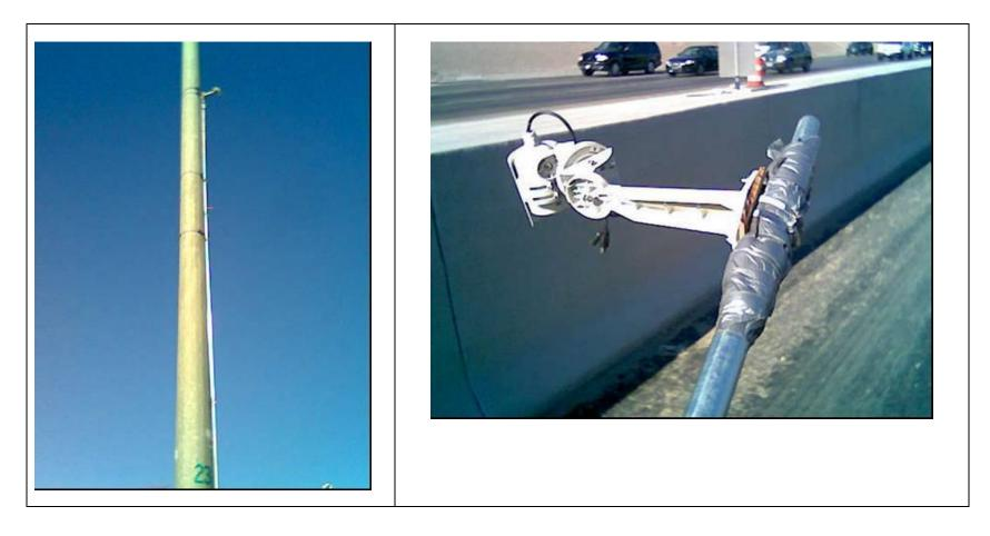
Figure 4.2 Camera Mounted on Light Pole 23 on I-15
