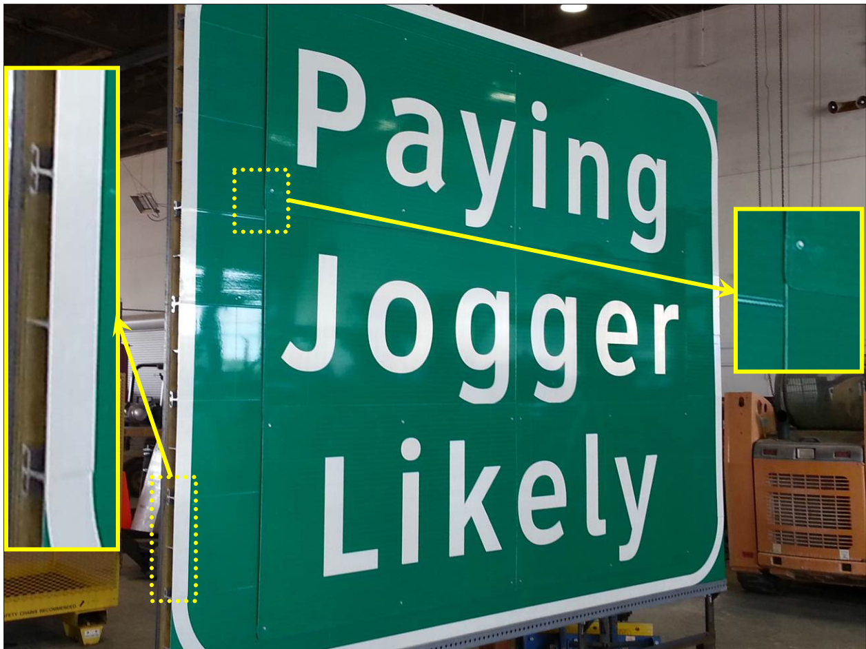
Figure 3.3. Overhead Guide Sign Construction.
