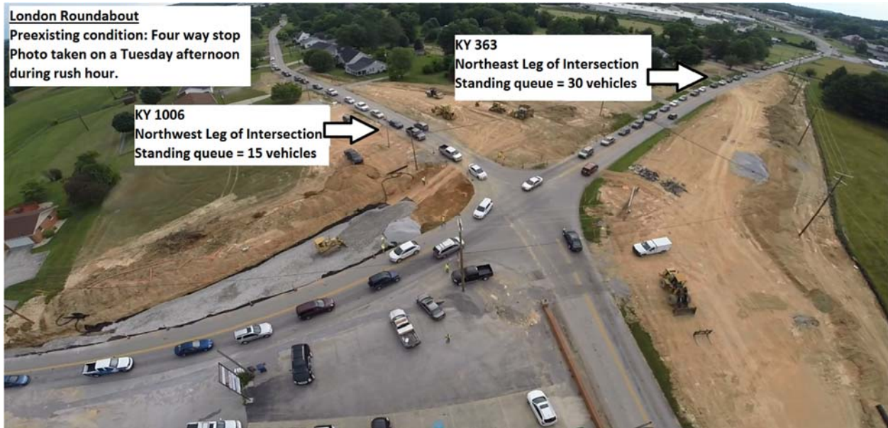
Figure 7 Queuing at KY 363 and KY 1006 When Connected by a Four-Way Stop Intersection
