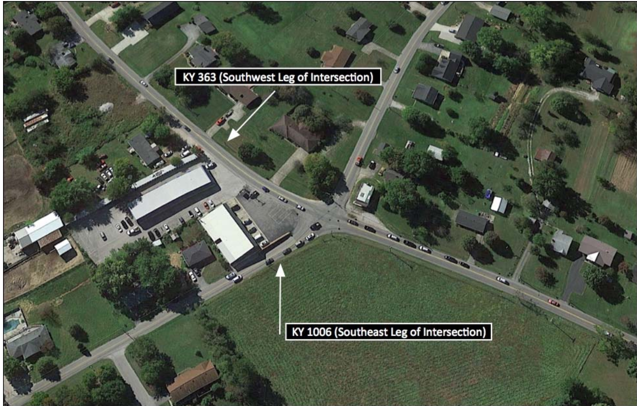
Figure 2 Aerial View of Four-Way Stop Intersection at KY 363 and KY 1006 Before Construction
