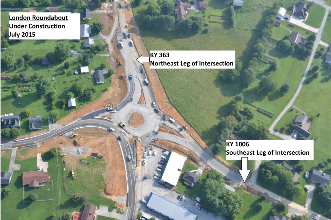
Figure 4 Aerial View of Roundabout During Subgrade Rock Placement
