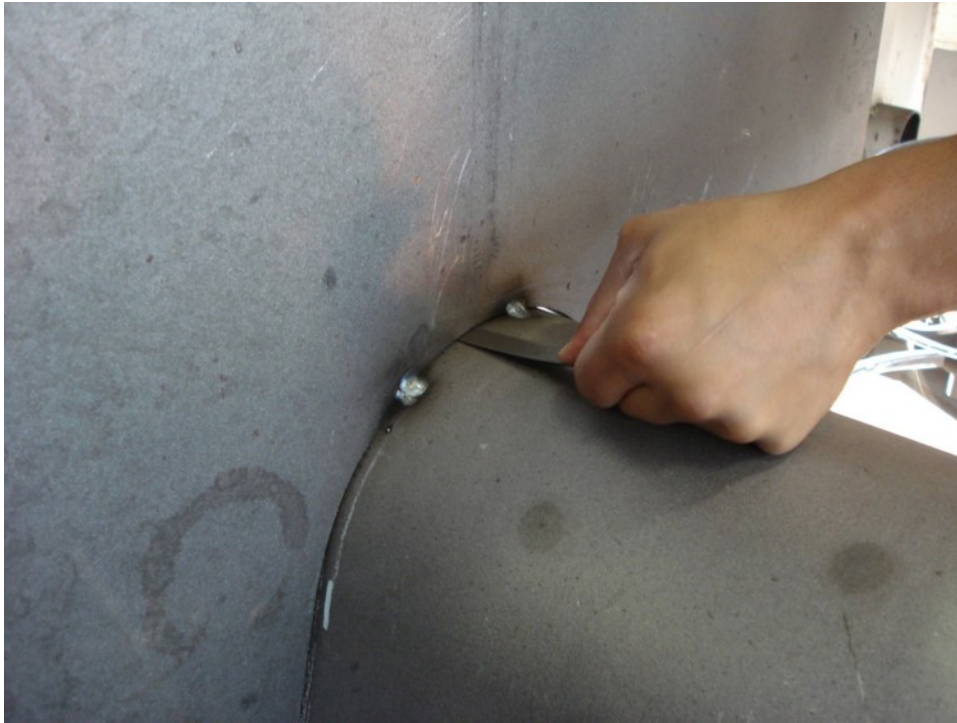
Figure 89. Extensive efforts for rib-to-floor beam fit-up
