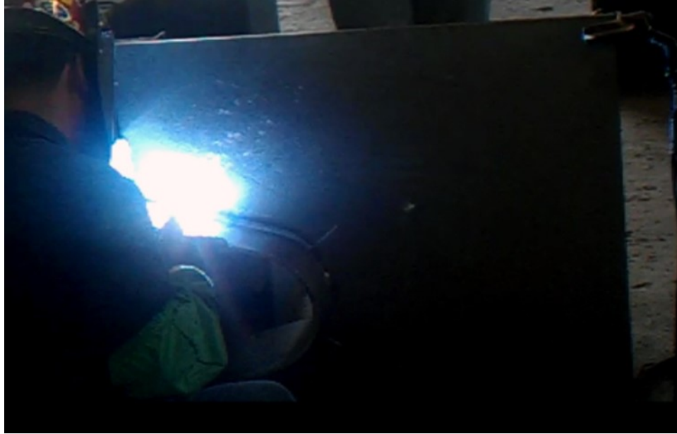
Figure 90. Manual welding of rib-to-floor beam connection
