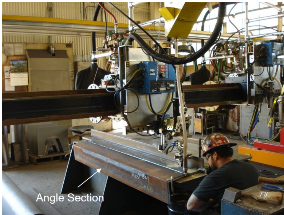
Figure 85. Modification of mockup specimen by addition of angle
