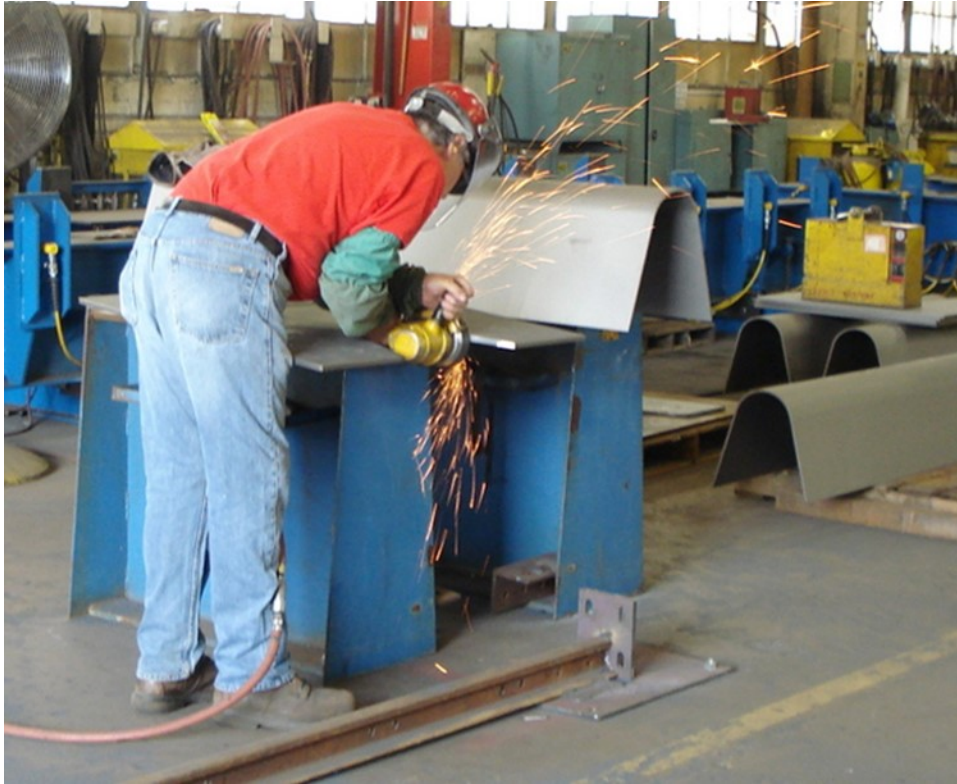
Figure 88. Grinding of floor beam to match with rib-profile
