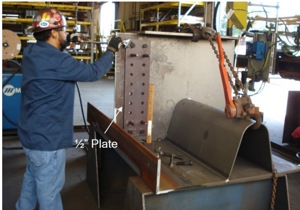
Figure 86. Modification of mockup specimen by splicing plate to floor beam
