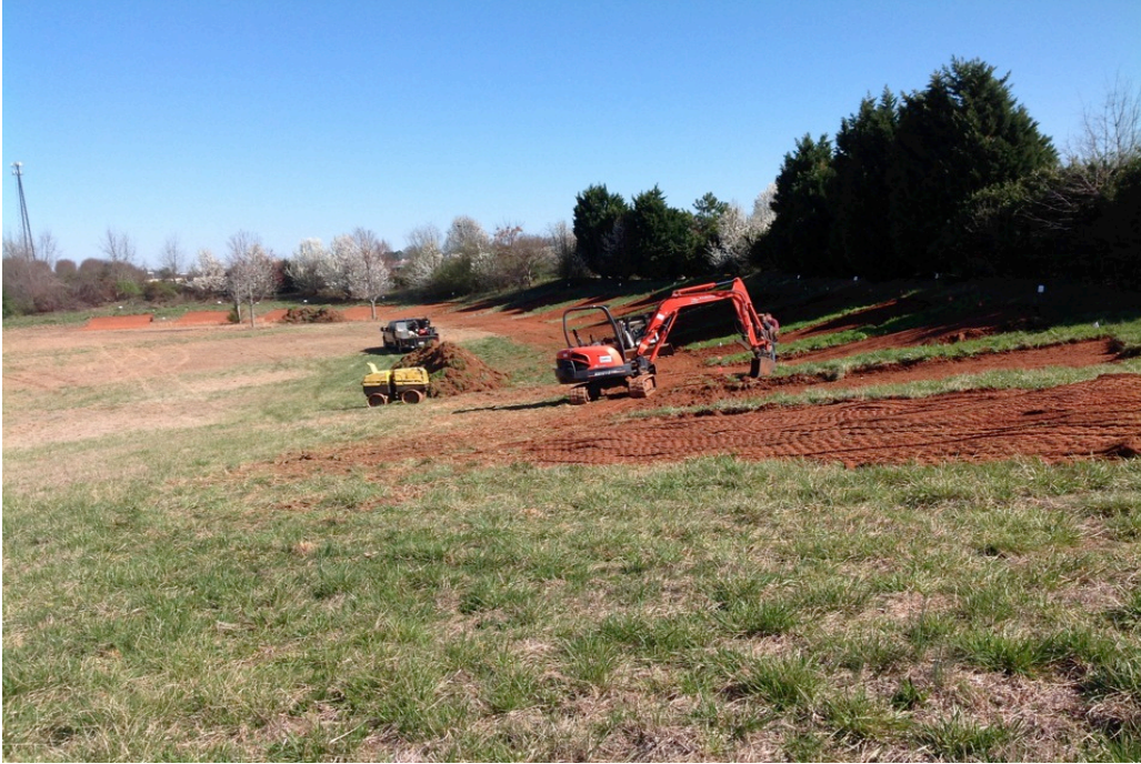
Picture 1. The construction of the plots on March 13, 2015 in Griffin, GA.
