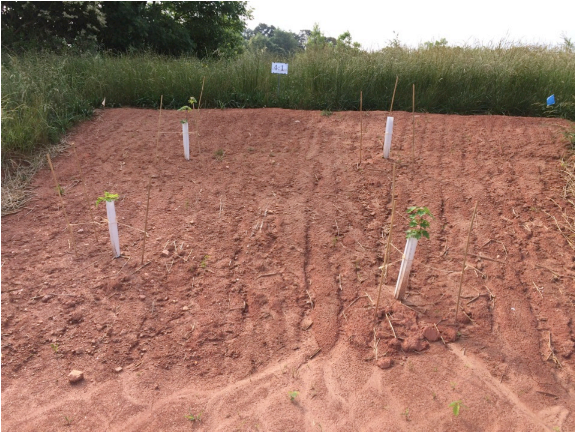
Picture 7. Erosion on May 20, 2014 after establishment on the 4:1 slope ration
