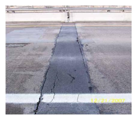
Figure 23 Bridge H-869E Pier 7 (breaking, joint debonding)
