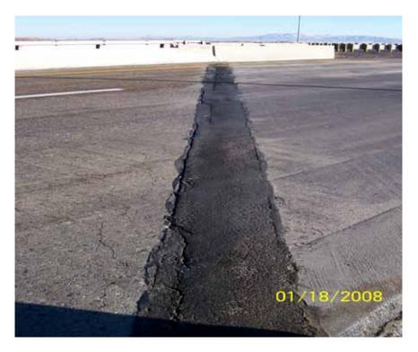
Figure 21 Bridge G-872 East Abutment (cracking, joint debonding)
