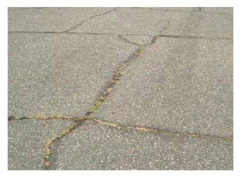
Figure 5 Reflective cracking
