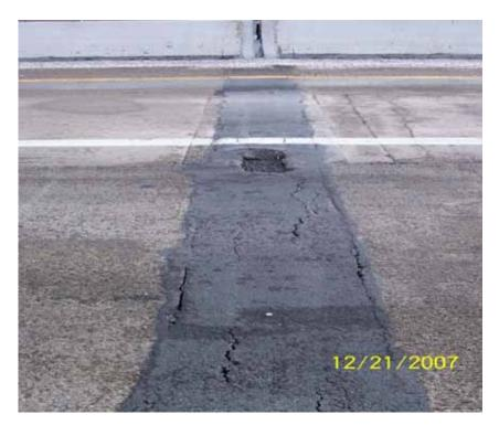
Figure 24 Bridge H-869W Pier 7 (joint debonding, pot holes, spalling)
