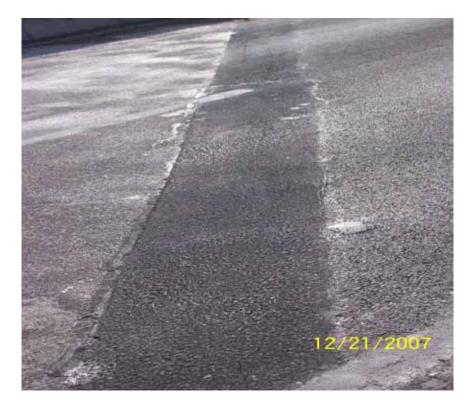
Figure 20 Bridge I-871 W East Abutment 2 (shoving)
