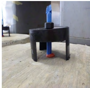
Figure 4.6: Downward installation of anchor
