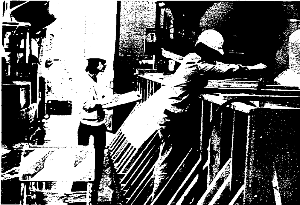
Figure 13. Taking soundings during break in concrete placement.
