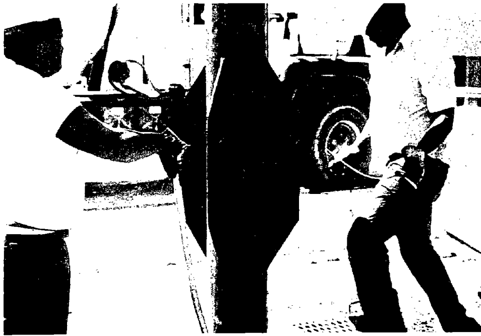
Figure 78. Fins added to tremie pipe to insure proper centering.
