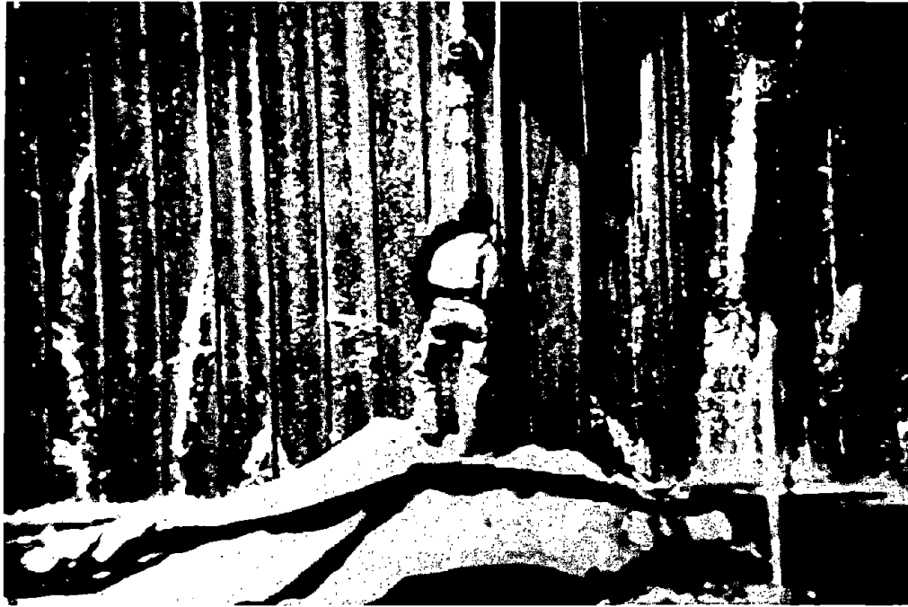
Figure 65. Mounding on surface of seal. This mound was located at one of the final tremie locations.
