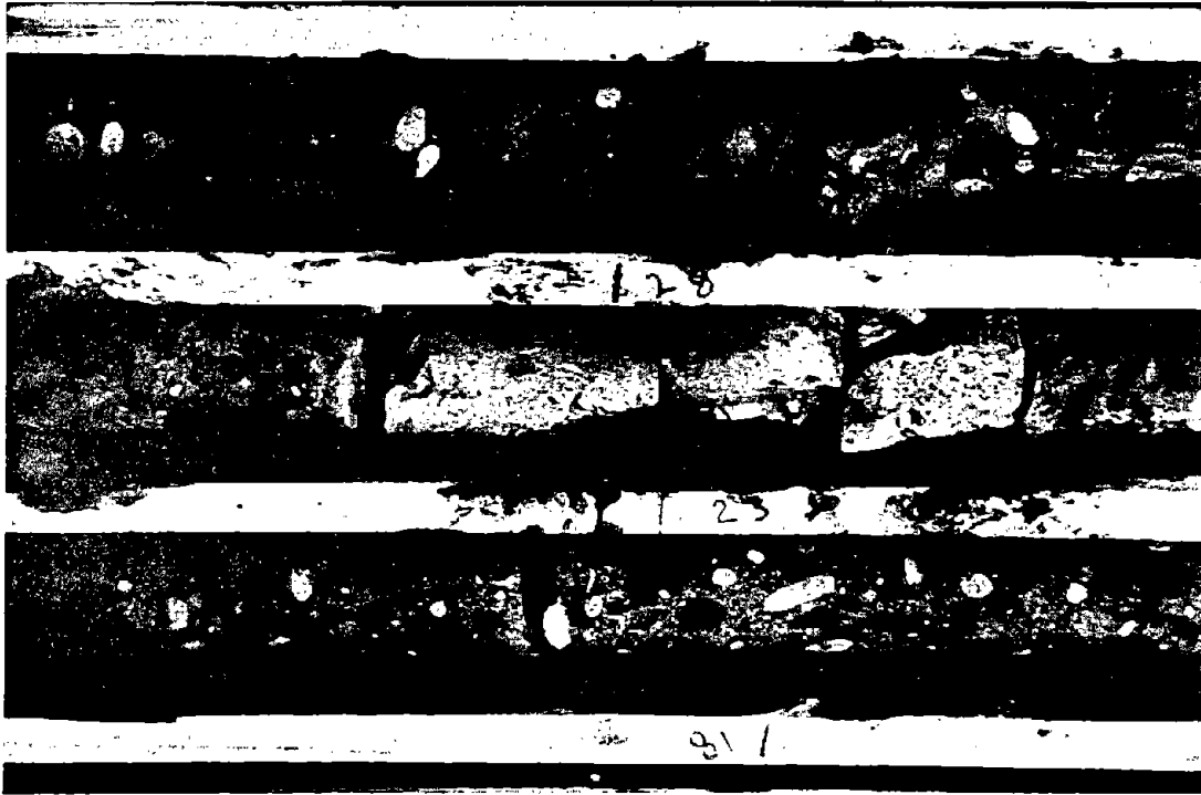
Figure 68. Section of core taken from tremie concrete. Note the area at the 23 ft (7.0 m) mark. This small zone of laitance was the worst concrete seen on the four cores.
