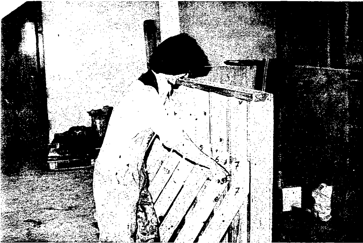
Figure 8. Partially assembled tremie placement box.
