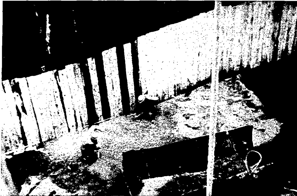
Figure 66. Low area in surface of seal. This photo was taken during preparation of the next lift of concrete.
