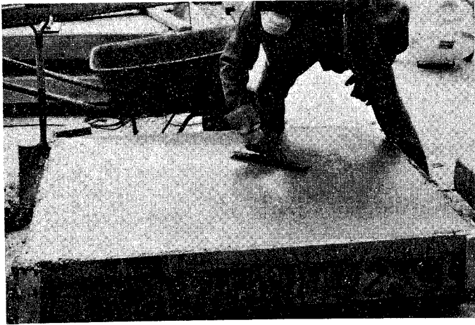
Steel trowel finishing of the "underlay" concrete
