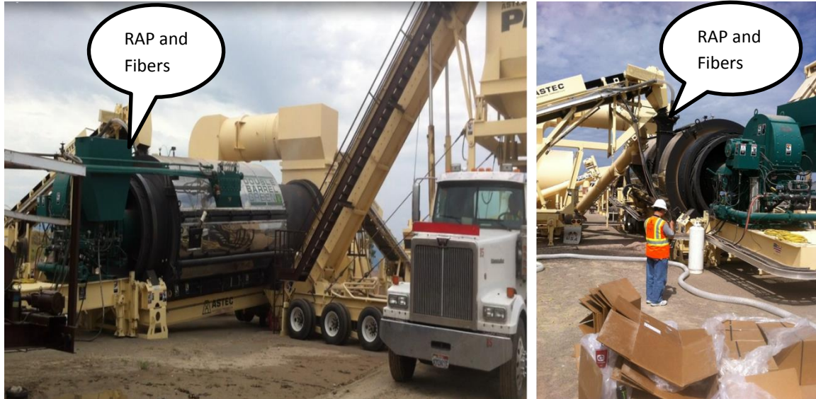
Figure 5. Process of Blowing Fibers into the HMA plant
