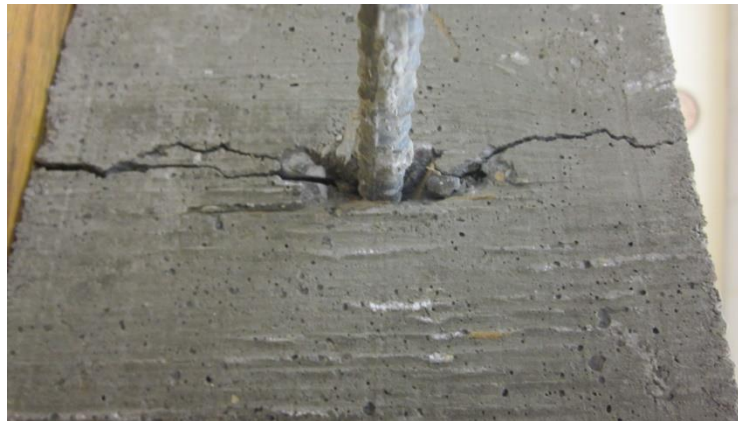
Figure 27: Typical Push Through Bond Strength Testing Failure Mode
