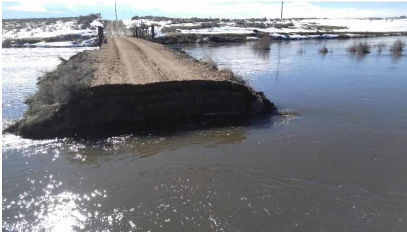
Figure 10. Camas Bridge May 2017
