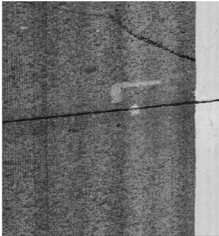
FIGURE 3-28 Marked measuring point in pavement surface laser data
