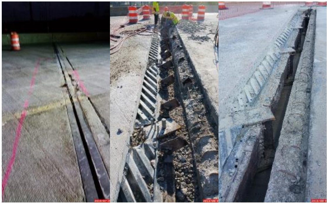
Figure: 26-28: Dam Demolition Progression from (a) Pre-Demolition, (b) after 4 Days of Demolition to (3) Pre-Construction Ready
