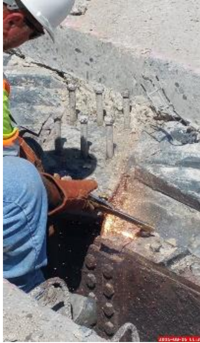
Figure 38: Torching and Removal of the Previous Metal Formwork
