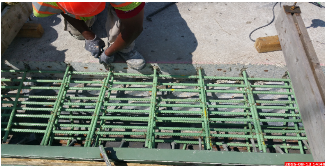
Figure 54: Implementation of the Stirrups and Rebars Through Tying
