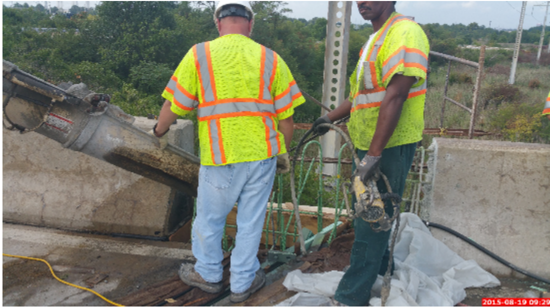
Figure 60: Filling of the Wing Wall and Parapet Base with Concrete
