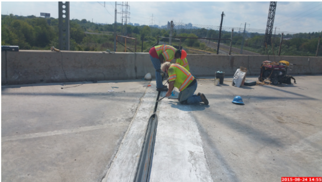
Figure 63: Implementation of the Strip Seal Extrusion into the Armoring
