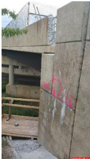
Figure 14: Wingwall, indicated by the Spray-Paint, to be demolished
