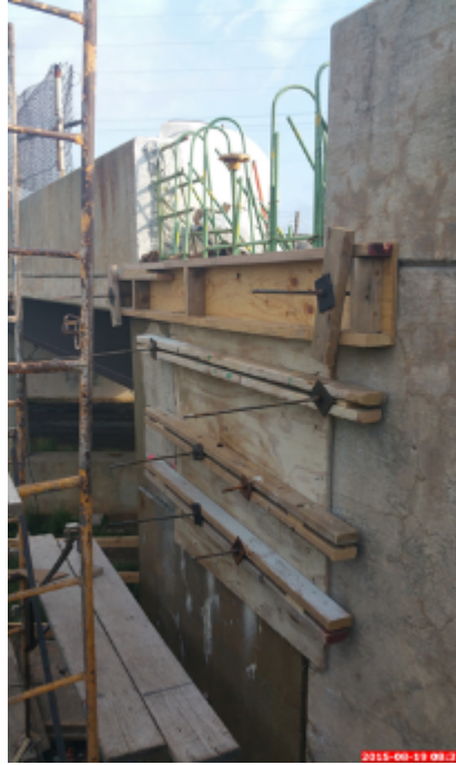
Figure 59: Formwork of the Wing Wall and Parapet Base
