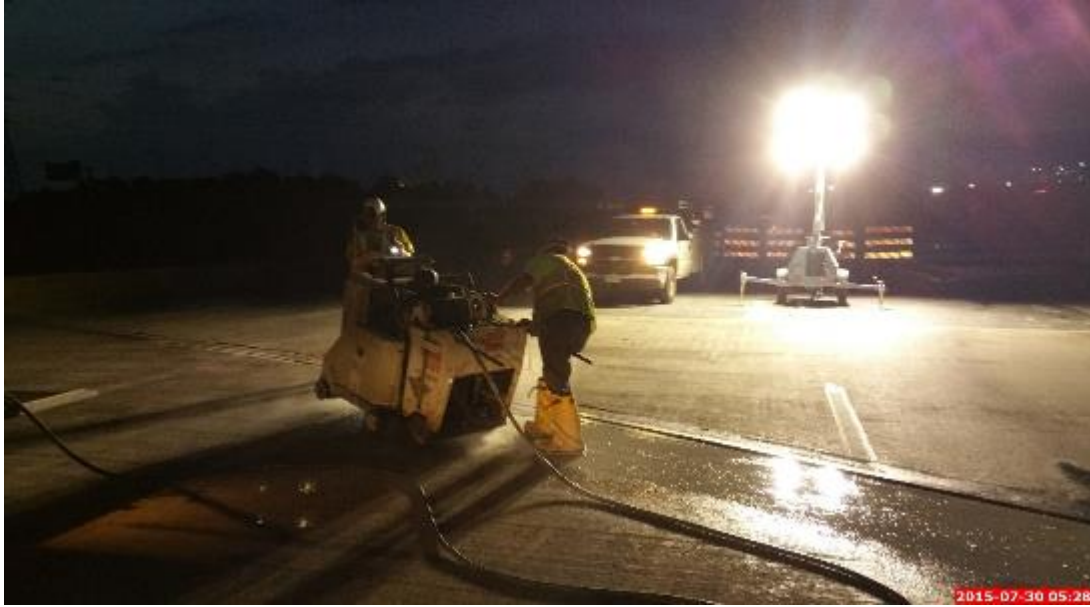
Figure 28: Pre-Construction, Deck Header Segmentation Through Concrete Saw Cutting with the Walk-Behind-Saw
