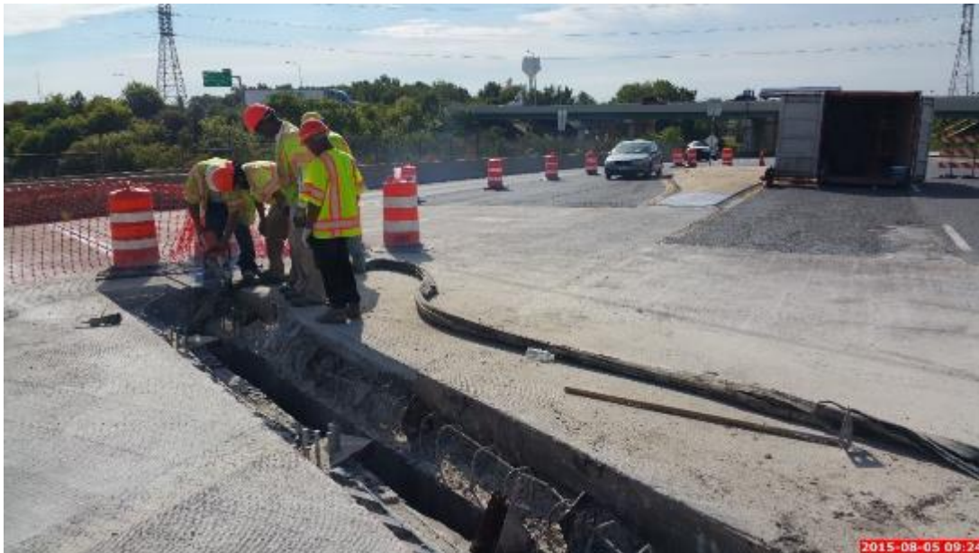
Figure 31: Removal of the Previous Cushion Joint Seal
