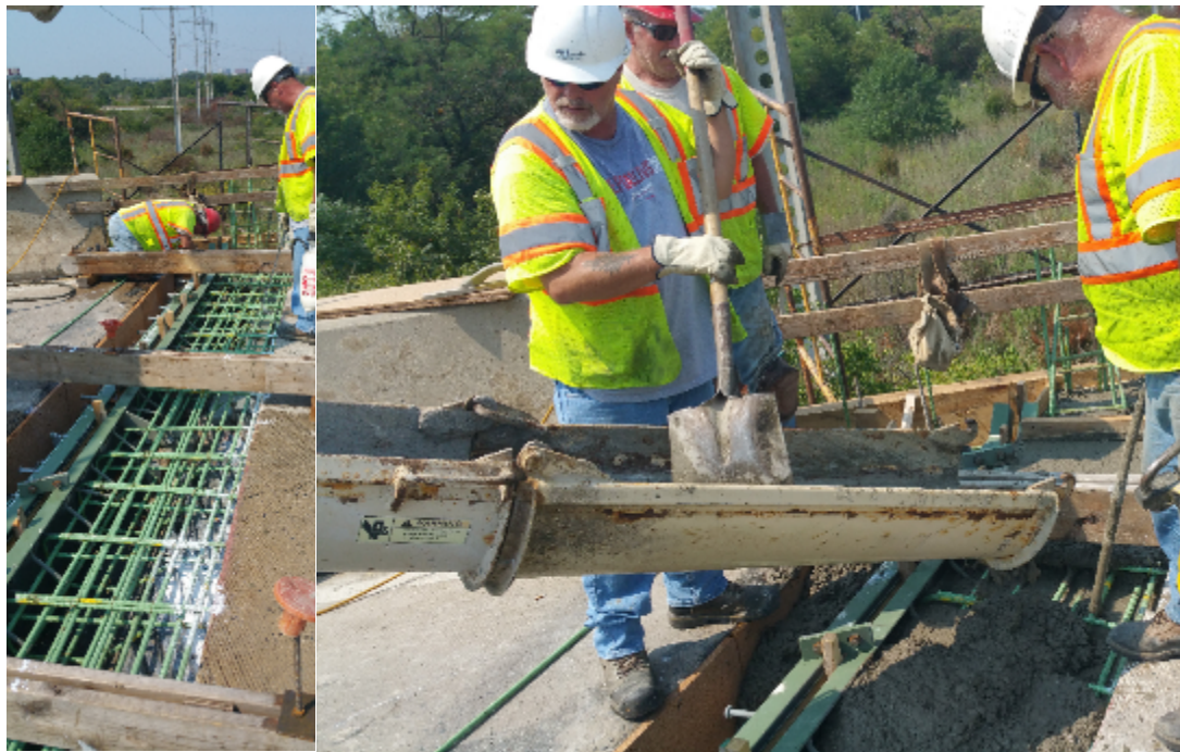
Figure 56: Preparing the Headers Before Pouring of the Concrete (a) Spraying of the Adhesive Spray and (b) During the Pouring with a Mechanical Vibrator Placed Within the Newly Poured Concrete to Facilitate Dissemination of the Concrete
