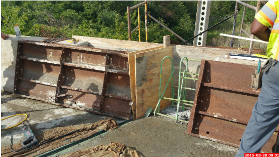
Figure 61: Formwork of the Parapet Bodies
