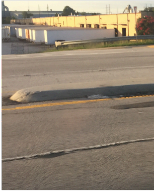
Figure 9-5. Raised Concrete Medians
