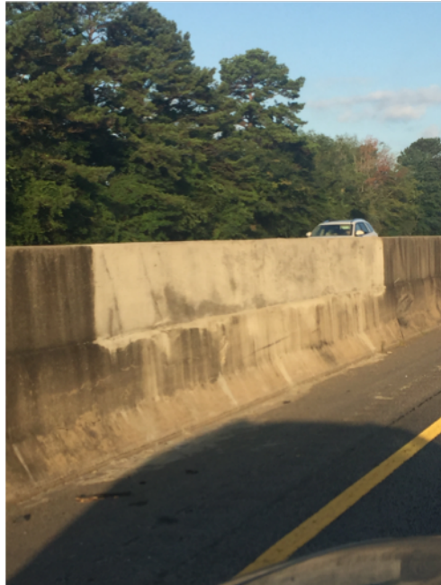
Figure 9-3. Repaired Glare Protection Concrete Sections on EB I-20
