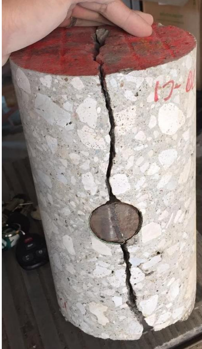
Figure 64 Tangential core collected over a dowel bar from WAY-30 at a location with a longitudinal crack. Note crack runs between aggregate above dowel bar, then runs through the aggregate underneath, indicating the concrete is stronger underneath.
