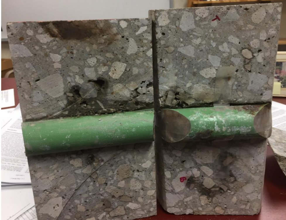
Figure 67 Two tangential cores collected at a joint on WAY-30, after sawing in half.
