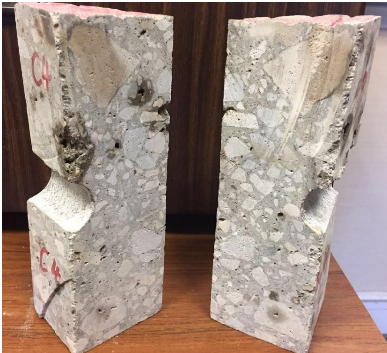
Figure 70 Slices from WAY-30 tangential cores showing more detail of entrapped air voids in area above dowel bars.
