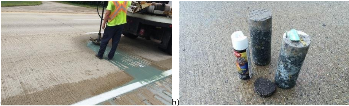
Figure 88 a) Core drilling on LAK-90, August 31, 2016; b) Concrete core samples.
