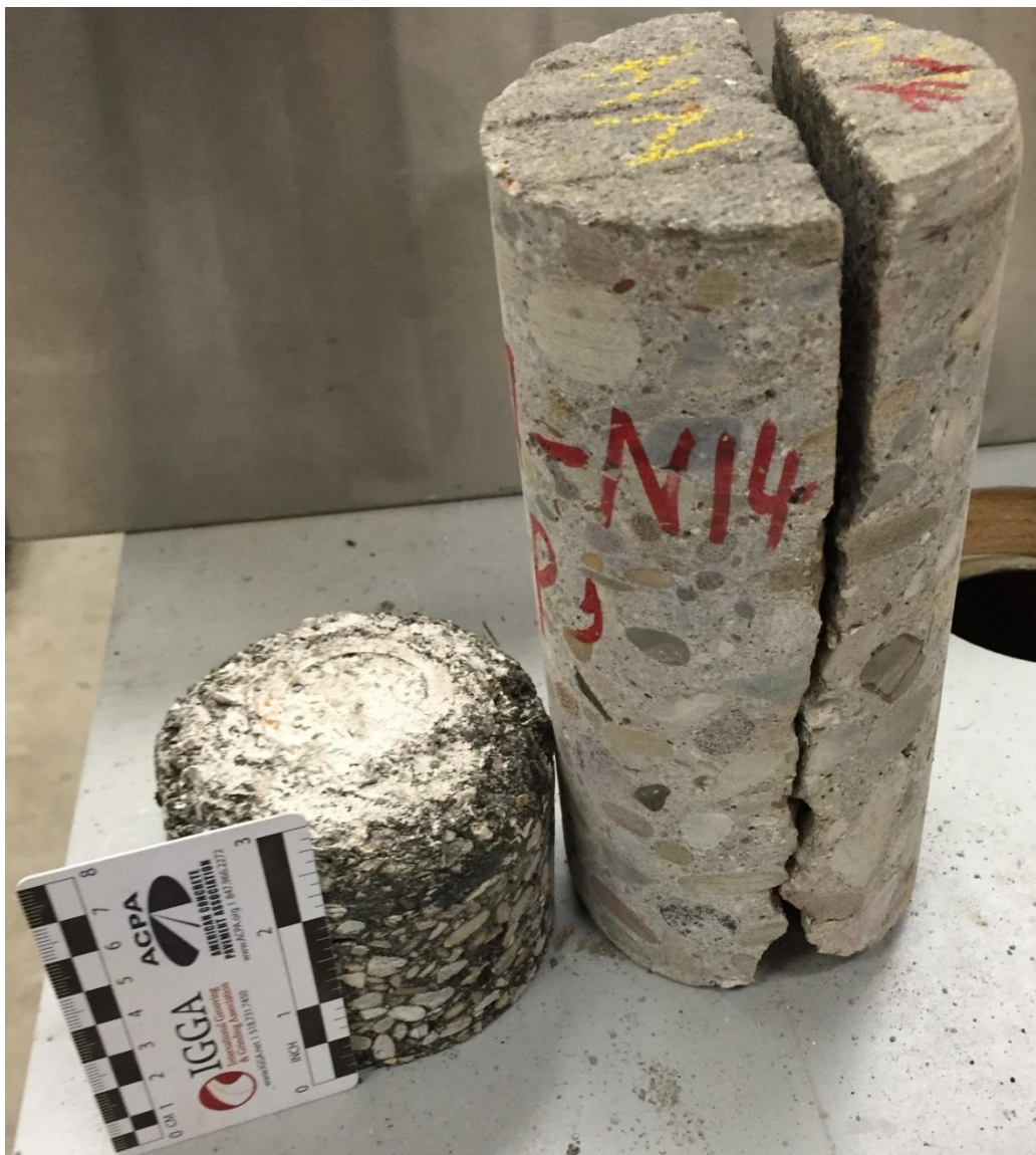
Figure 71 Core collected at a joint on WAS-NOB-77 northbound.
