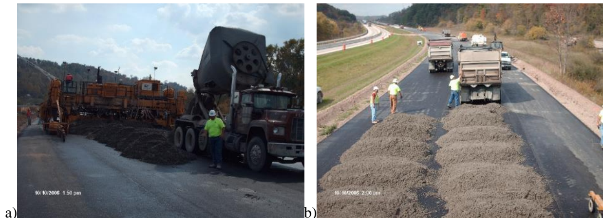
Figure 50 Wetting the bondbreaker before placing concrete. Photos dated Oct. 10, 2006.
